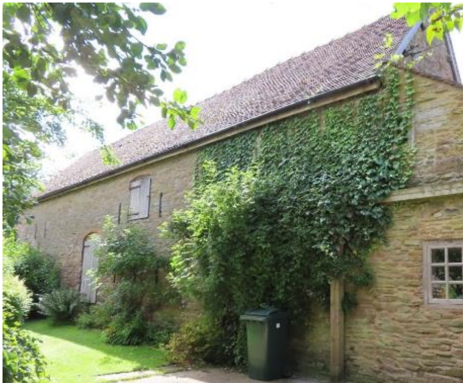
Photograph 4. Buildings at Church House Farm. Exterior.
