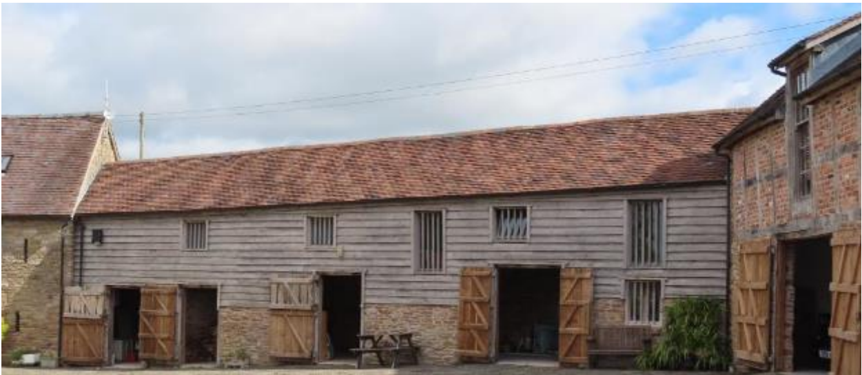
Photograph 2. Buildings at Church House Farm. Exterior.
