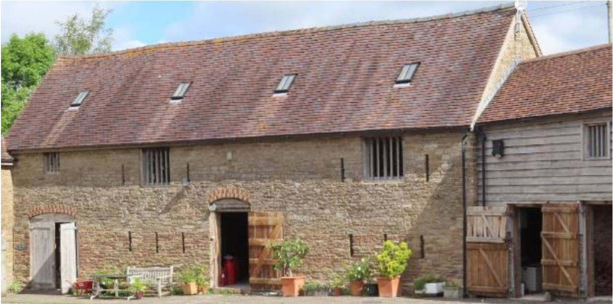
Photograph 1. Buildings at Church House Farm. Exterior.
