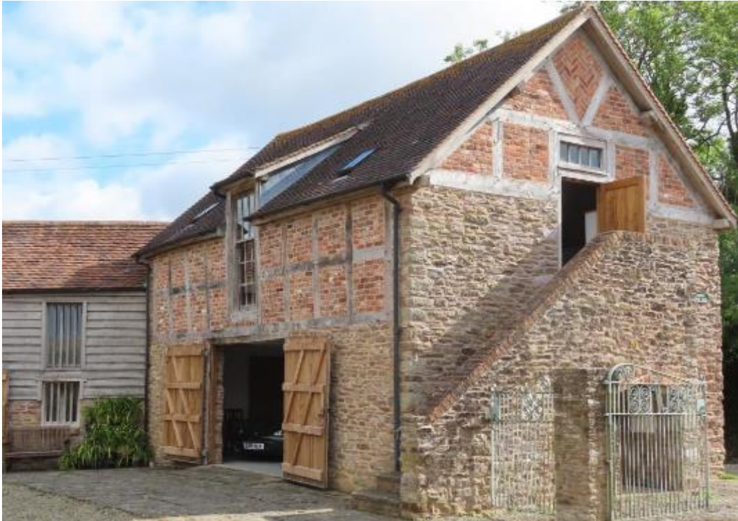
Photograph 3. Buildings at Church House Farm. Exterior.
