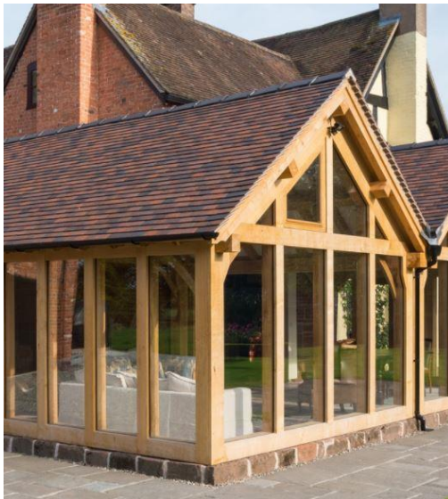
Figure 13.0 – Example of Glazing panels set into Oak frame (Copyright Shropshire Oak Carpentry Company)
