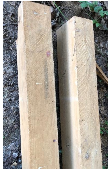
Figure 4.0 – Example of milled Oak for use in the timber frame
