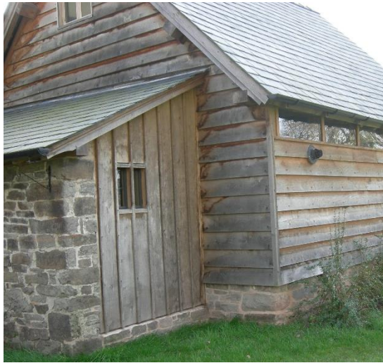
Figure 5.0 – Example of wooden cladding above stone plinth
