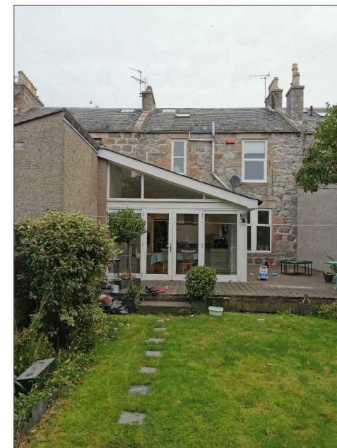
Photo of Existing South Elevation
