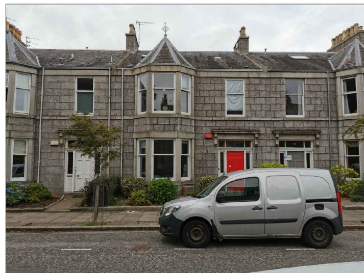
Photo of Existing North Elevation
