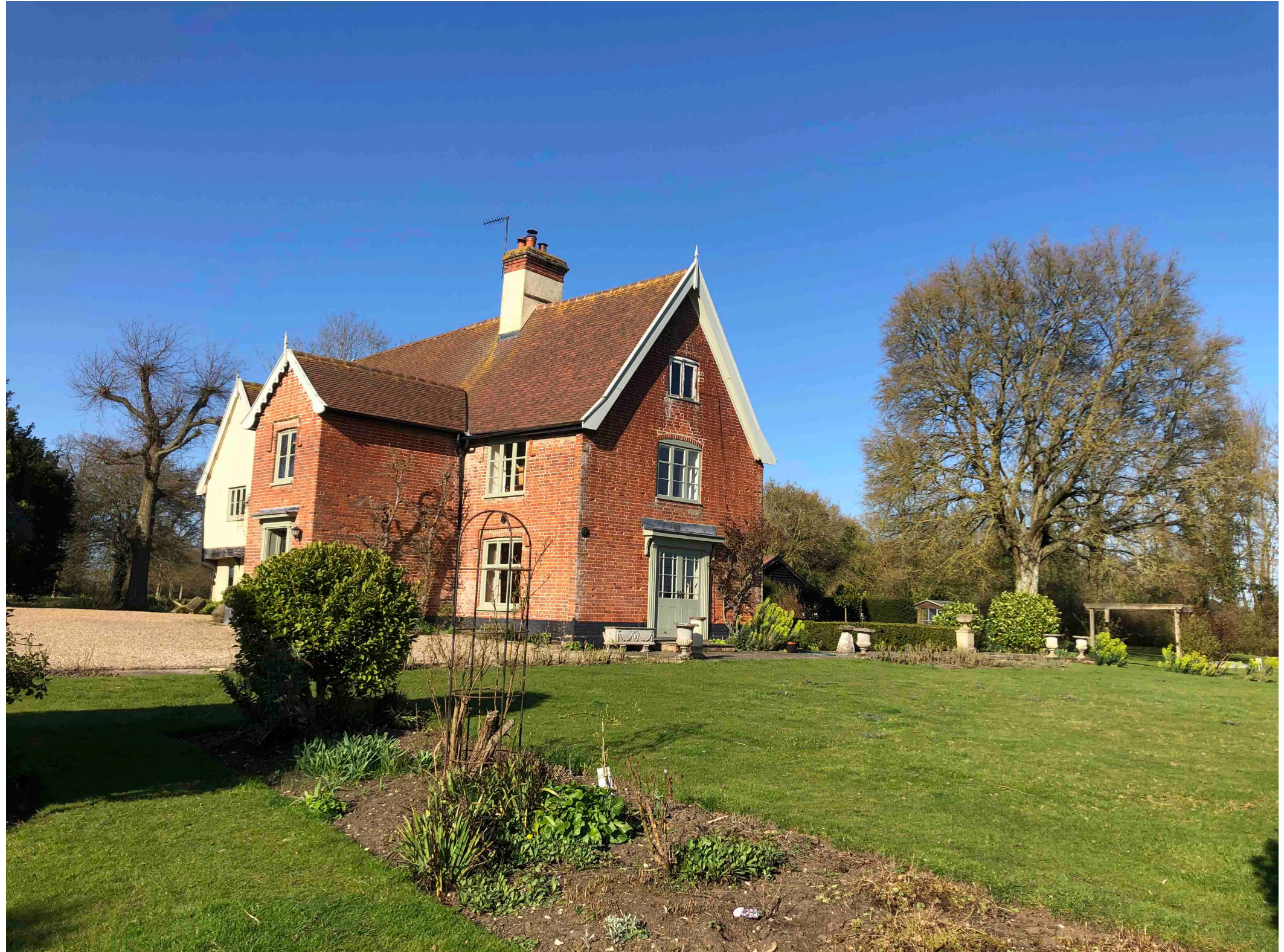
South West view. Extension will be recessed back and largely hidden. You can just see the garage block which the extension will link with.
