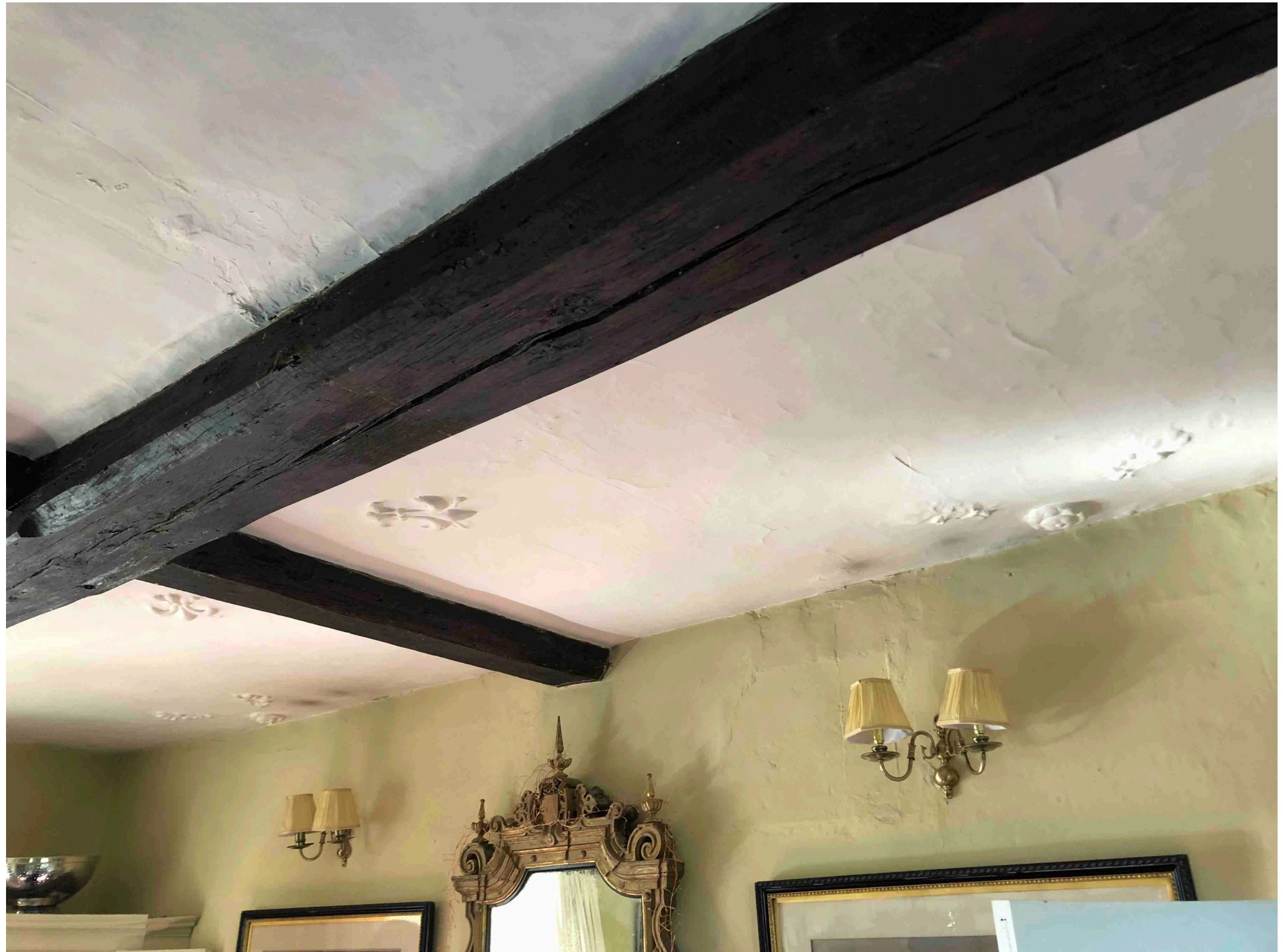
Internal view of drawing room showing ceiling motifs and wall believed to have been inserted in 1920's that artificially subdivides space. Motifs continue beyond wall
