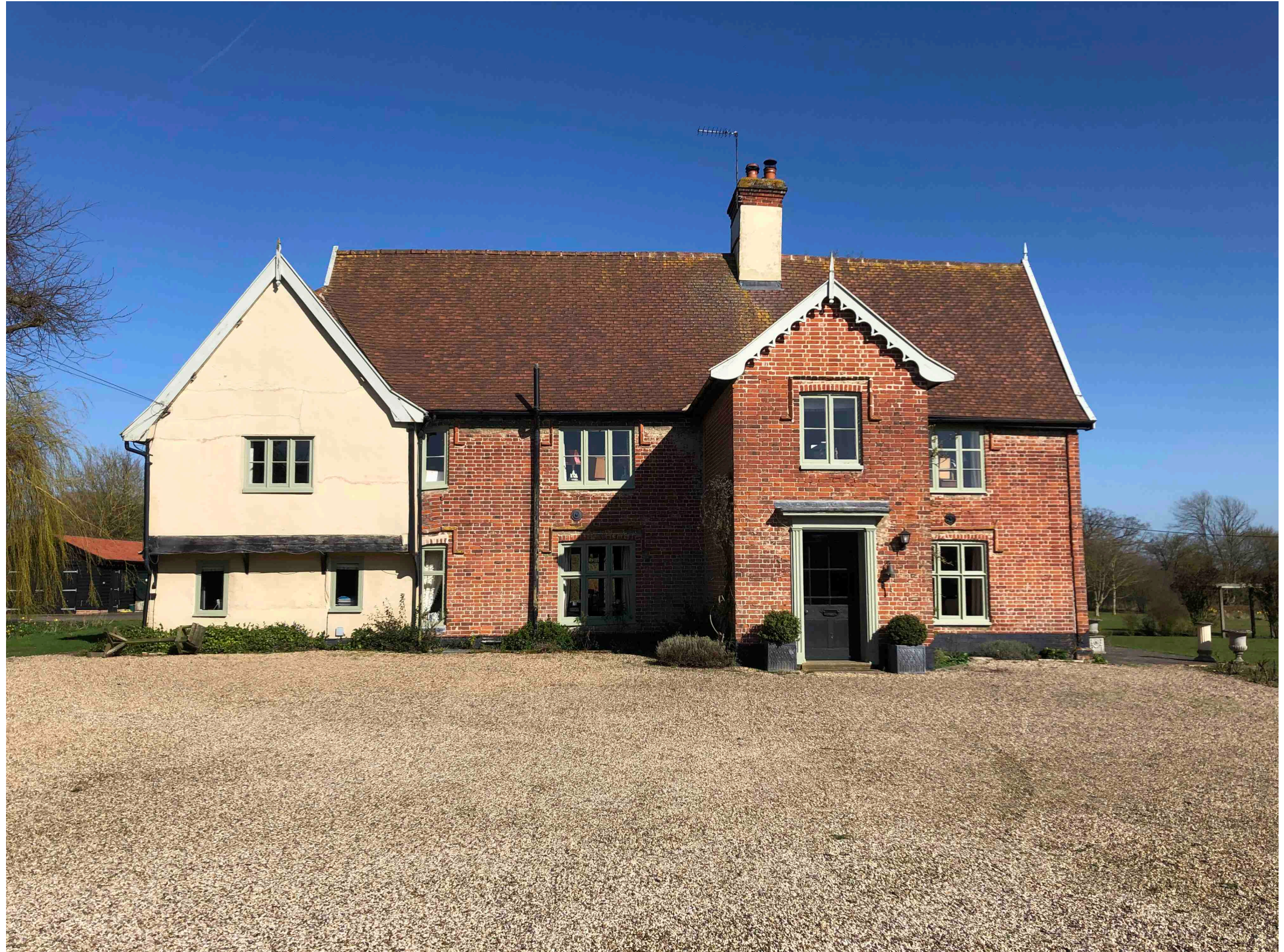
Front elevation. Driveway has moved but the front remains unchanged. Rear extension will be unseen.
