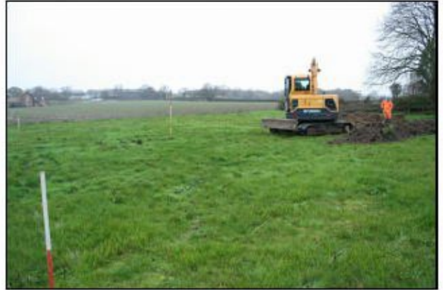
2 View of site looking south-east before excavation of trenches
