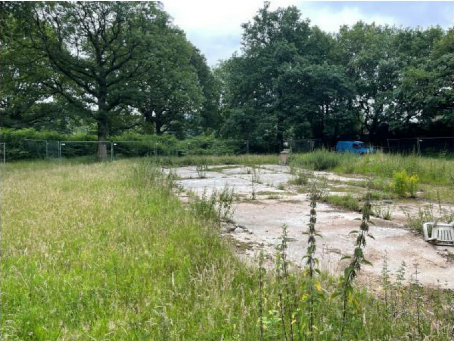
Photo 2: Showing the concrete slab
