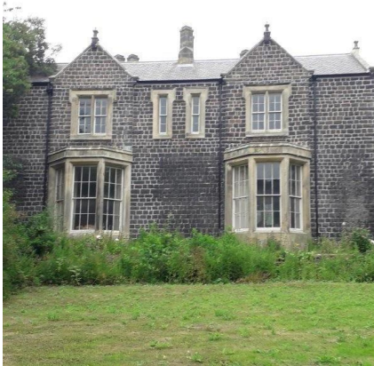
The West elevation on completion
