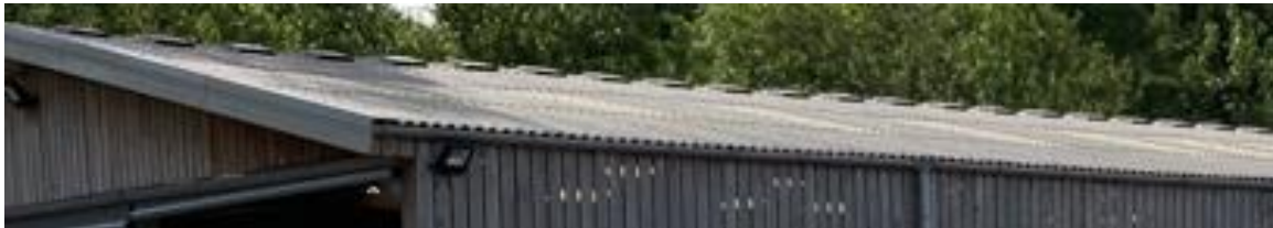
Photo 4 (Indicates the roof covering of one of the existing agricultural buildings)
