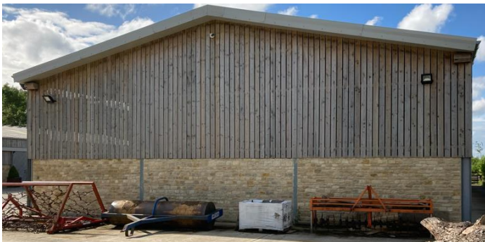
Photo 1 (Existing building at Grove Park)
