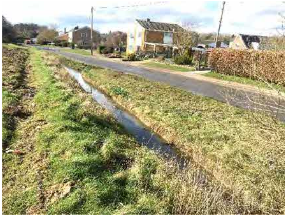
Photograph 3. Western end of ditch along northern Site boundary, adjacent to Forest Road. The ditch had recently been dredged and banksides cleared of vegetation.
