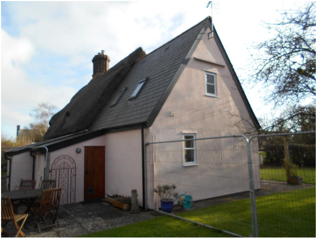
3. Calford Green Cottage - view of West side and part rear elevation
