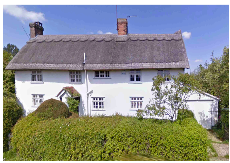
STREET VIEW SOUTH ELEVATION AS EXISTING
