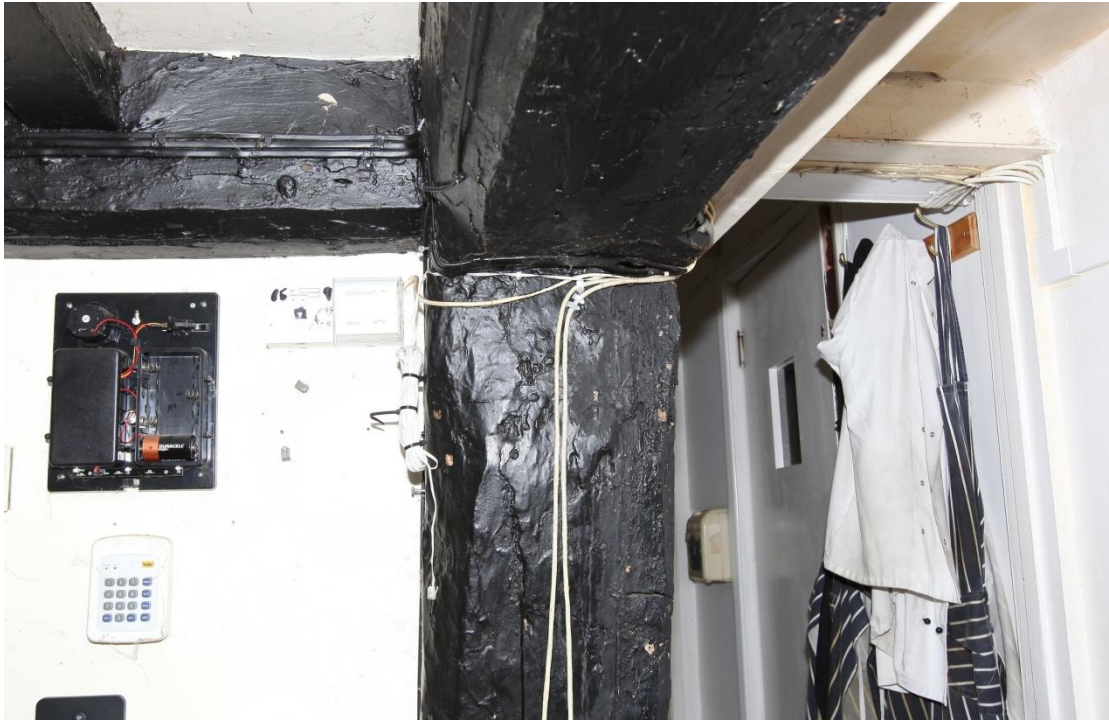
Illus. 11. A detail of the rear storey post to the left in illus. 9 showing what may be the outline of a carved capital with an attached shaft beneath. The carving has been cut away and the surface is now concealed by thick filler of some kind but it may repay careful investigation.
