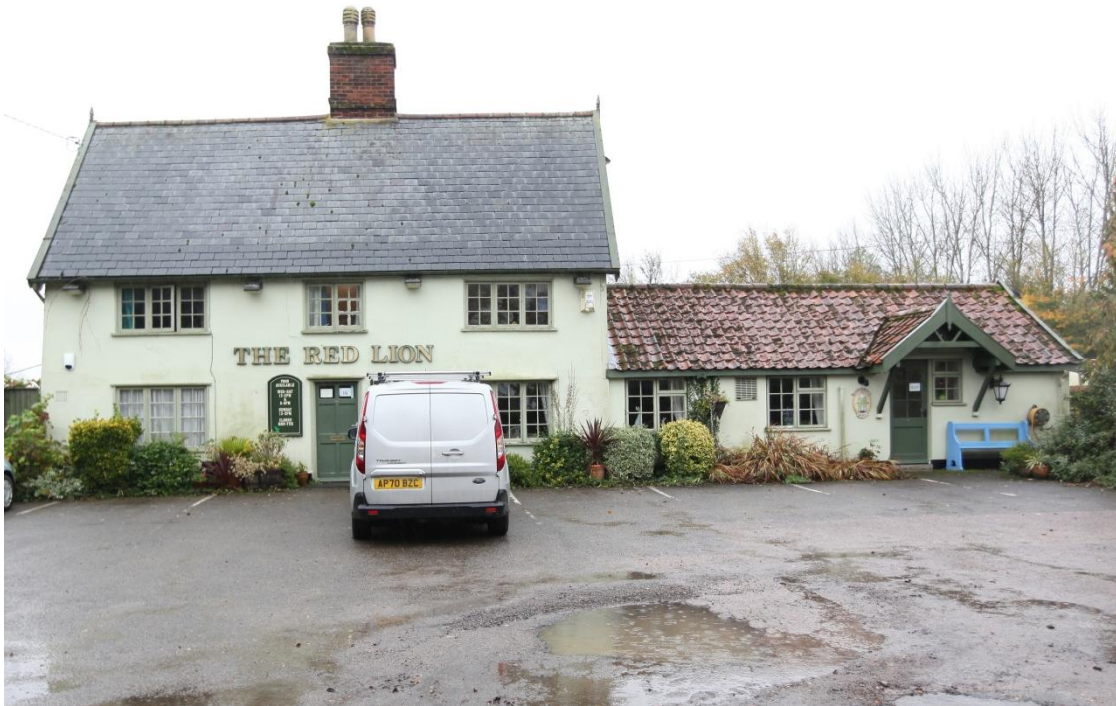
Illus. 1. The northern facade which in its present form is likely to date from the building's conversion into a public house in circa 1880. The decorative Mock Gothic barge boards, the brickwork of the chimney and the casement windows are typical of that period. In 1964 the single-storied range on the right terminated at a chimney in the position of its hooded entrance and has since been either extended or rebuilt (figure 7).
