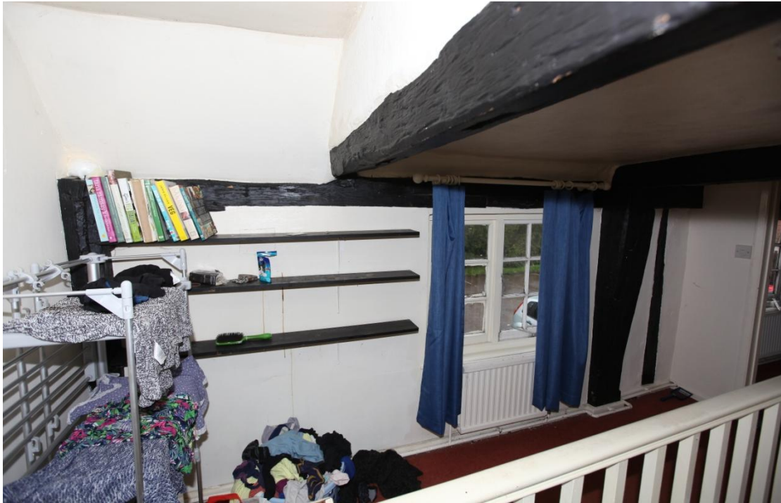
Illus. 19. The front wall showing the first-floor window above the present central entrance door with the jowled storey post of the missing partition on the left. The jowl contains a mortice for a wall brace which is lacking from its rear counterpart (illus. 16) suggesting an internal door lay against the back wall. The tie-beam in the centre contains empty stud mortices and formerly connected these storey posts.
