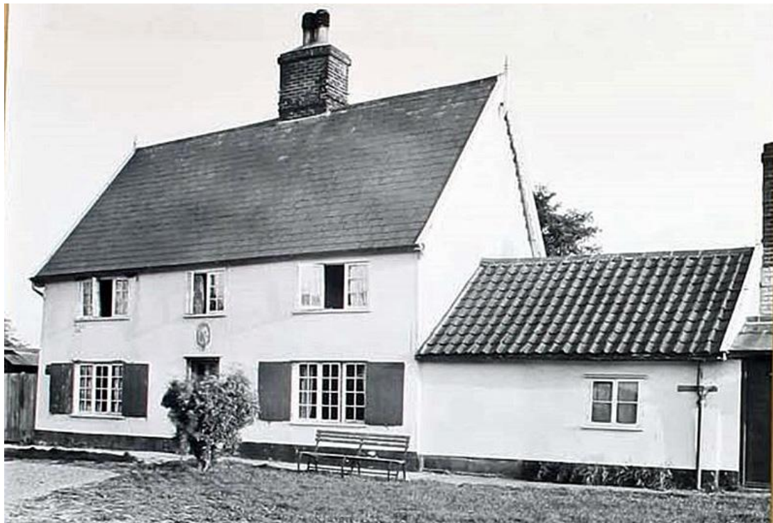
Figure 7. A photograph of 1964 (Royal Commission Archive). The single-storied shed probably dated only from the early-20 th century as its facade was not indented as in figures 4-5. It has since been extended significantly and possibly rebuilt.
