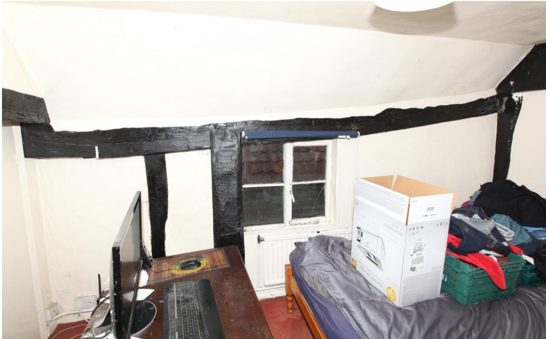
Illus. 17. The rear wall of the bedroom above the bar with the western gable on the right. The jowled storey post to the left of the present window adjoined a missing partition that divided the two-bay hall chamber on the left from the small parlour chamber on the right. The tie-beam of this partition now adjoins the chimney to the left. An identical partition would have existed on the ground floor. Note the 16 th century-type edge-halved and bridled scarf joint in the roof-plate above the exposed stud. A large gap in the frame extends from this stud into the cupboard behind the chimney and indicates the position of the 16 th century chimney (i.e. against the back wall of the high-end bay).
