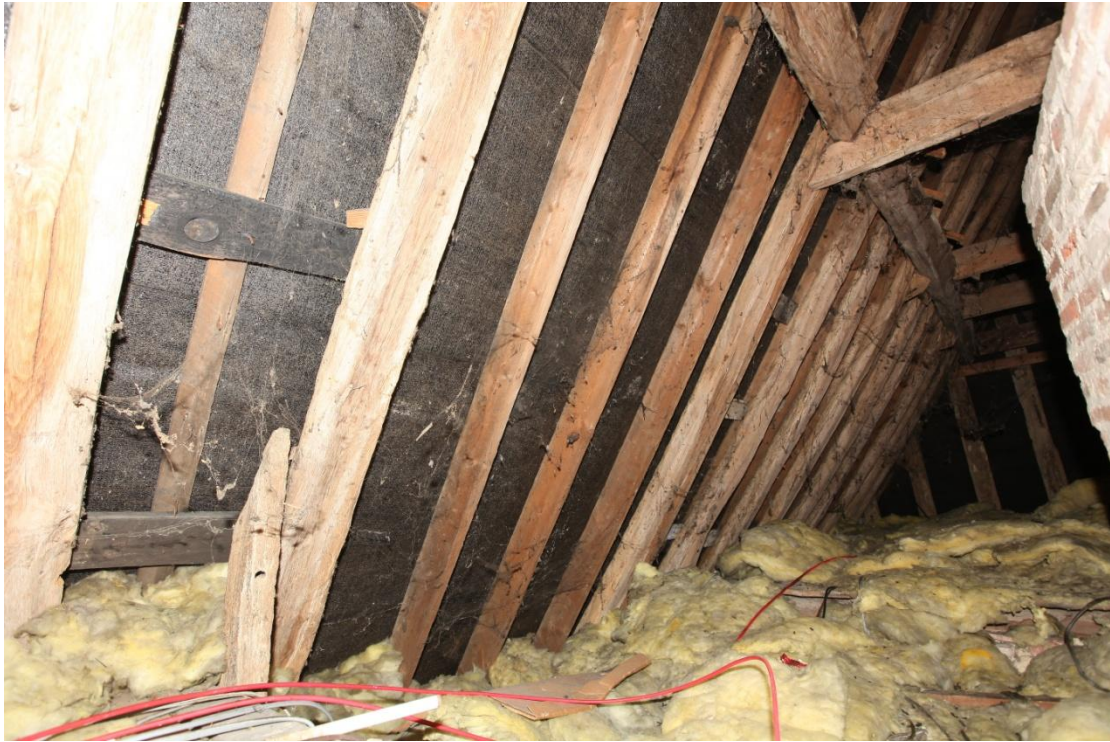
Illus. 21. The front of the roof structure with the chimney on the right. Unusually there is no evidence of any other wind bracing, whether nailed or pegged. Note the three pine rafters adjoining the stack in the centre which are late-19 th or 20 th century replacements.
