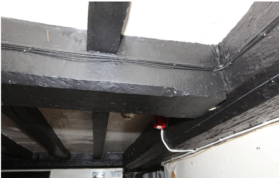
Illus. 10. A detail of the typically 17 th century curled 'lamb's tongue' chamfer stop to the living room's axial joist. The square or slightly tall-sectioned common joists indicate a date in the second half of the century. The axial joist overlaps the deep chamfer on the earlier binding joist to the right which contains mortices for original flat-sectioned common joists (one of which is visible at top right).
