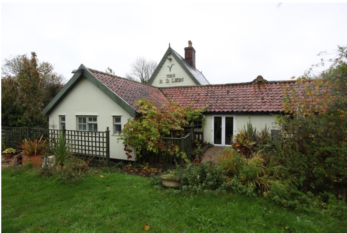
Illus. 2. The building from the west showing the modern single-storied additions in the foreground. These were not present in the 1970s and probably date from the 1980s as they appear to be mentioned in the 1988 listing description.
