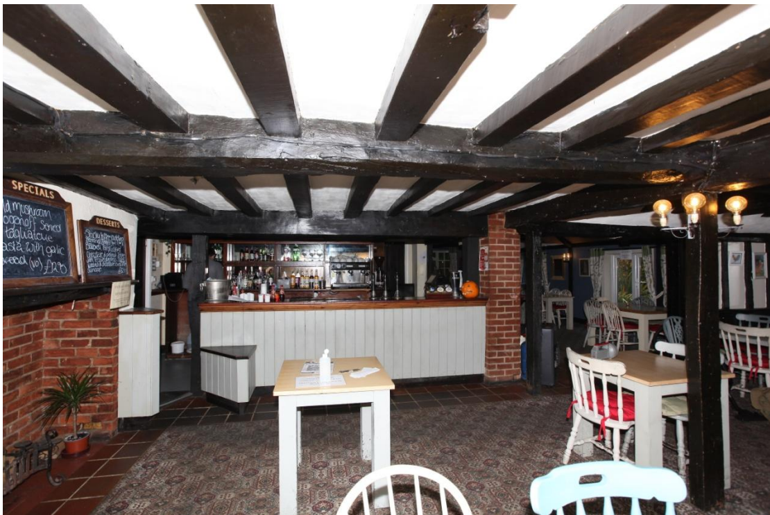
Illus. 4. The bar area seen from the north, with the rebuilt 20 th century fireplace in the 17 th century central stack on the left. The ceiling is a 17 th century replacement supported by the chimney and there is no trace at this level of the original partition that divided the 16 th century hall from its small parlour. The mid-rail to the right contains empty mortices for the western gable studs which have also been removed and the timbers in the single-storied extensions beyond are late-20 th century Mock Tudor insertions.
