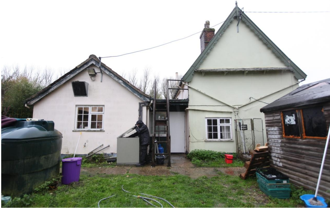
Illus. 3. The eastern gable with its traditional drip board and decorative Victorian barge-board. The steep pitch of the roof indicates it was designed for thatch and its present slate probably dates from the building's remodelling in circa 1880. The parallel outbuilding on the left is a recent addition that was not present in the 1970s.
