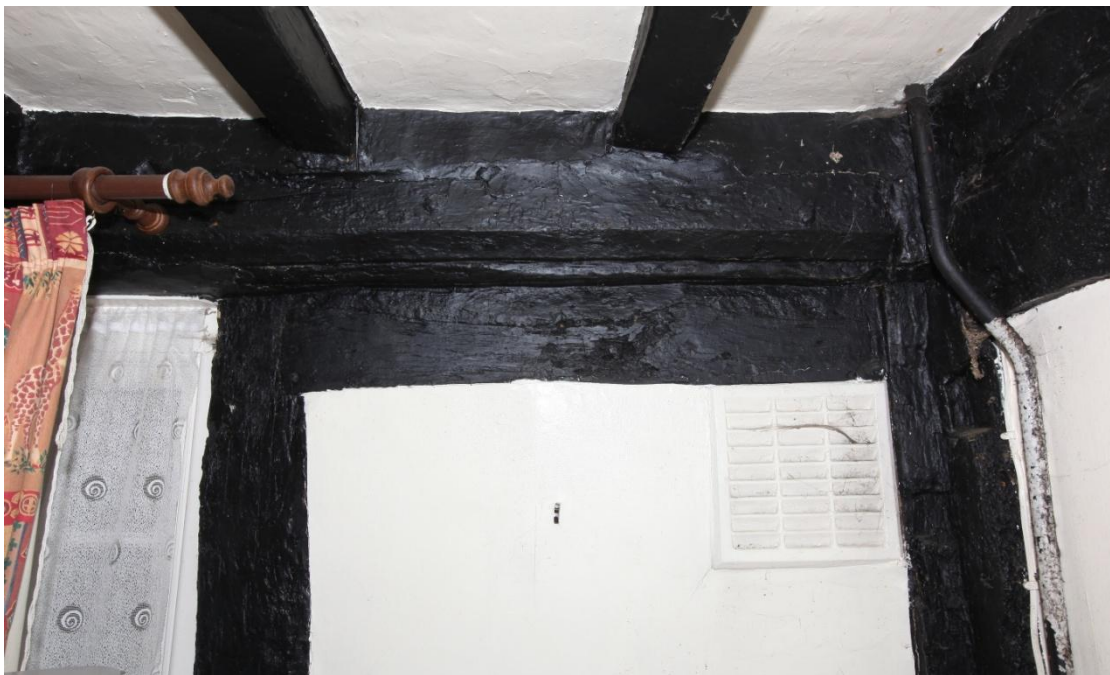
Illus. 8. A detail of the blocked door that almost certainly opened onto the original cross-passage. The lintel is a nailed insertion and the mid-rail is largely hidden by a pegged and chamfered clamp (rail) that supports the 17 th century ceiling joists. This door is likely to have served one of the two cottages until circa 1880.
