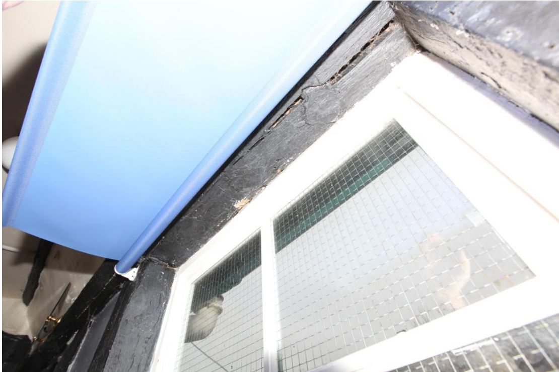
Illus. 14. A detail of the rear roof-plate to the left in illustration 13 showing three distinctive diamond-shaped mortices for 16 th century window mullions.
