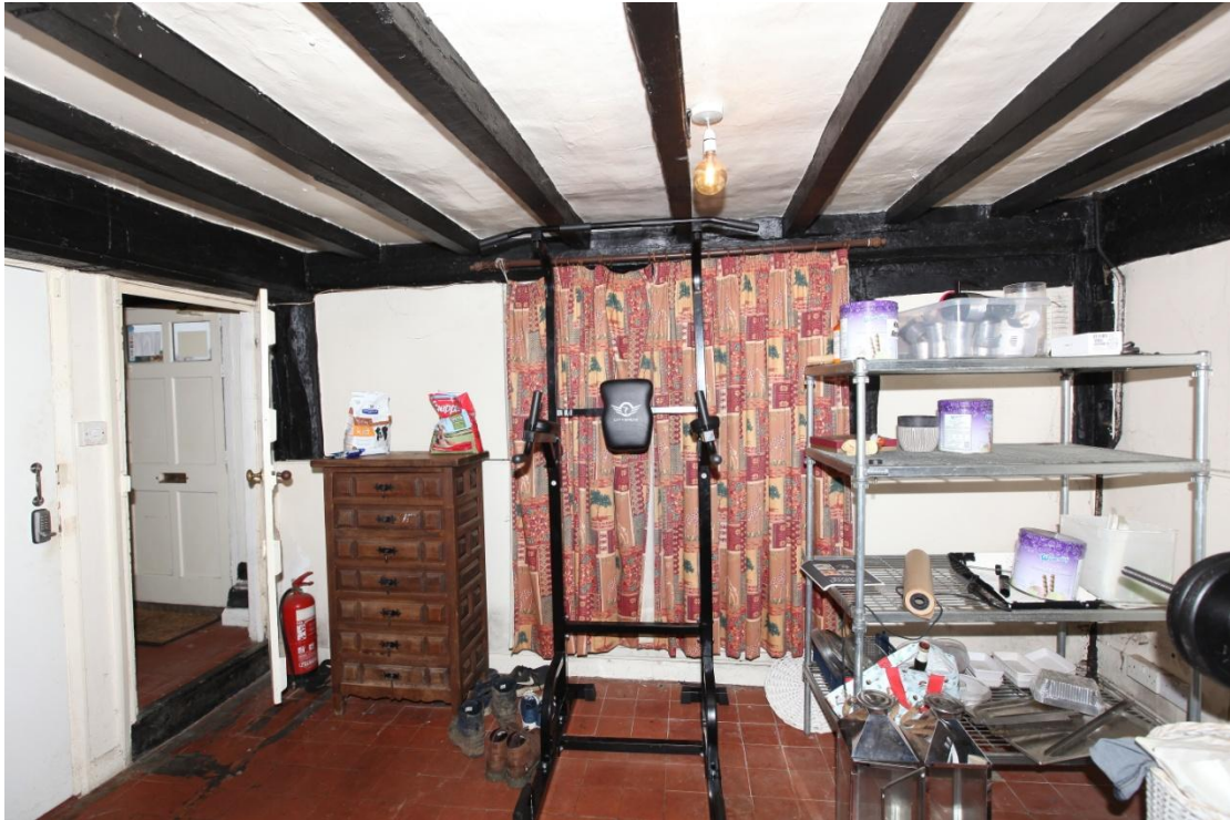
Illus. 7. The front wall of the living room (as labelled in figure 9) with the entrance on the left. As in the bar area the ceiling was rebuilt after the chimney's insertion and the 16 th century binding joist above the doorway to the left contains mortices for the original longitudinal joists. The position of the 16 th century entrance is indicated by the nailed lintel to the right (illus. 8). The mortice pegs in the exposed mid-rail of the eastern gable on the extreme right are hidden by thick paint and filler, but this timber is likely to contain evidence of central doors that opened into the missing service bay.
