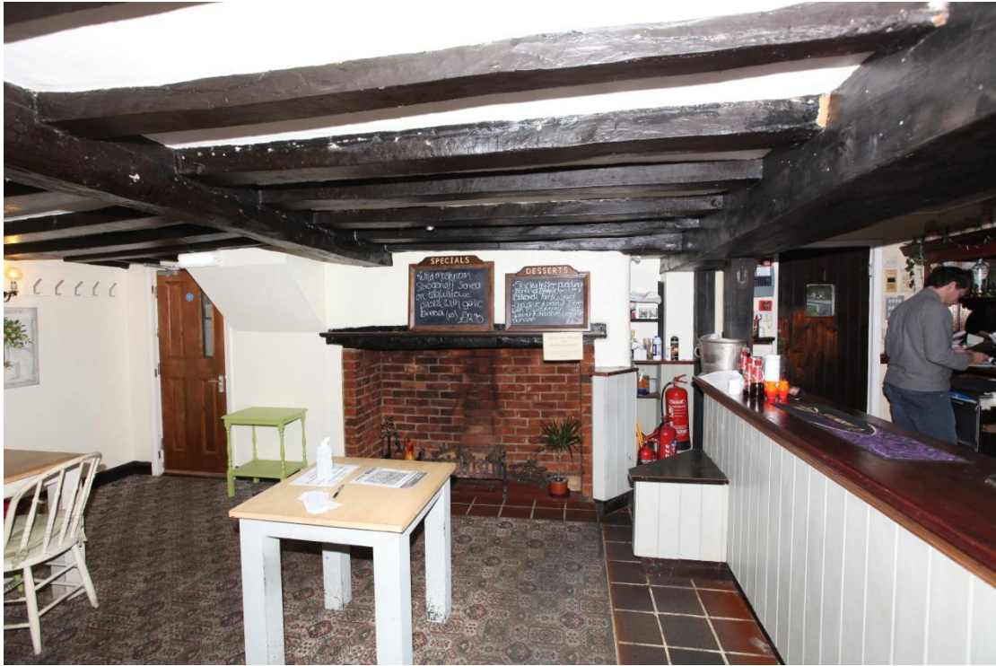
Illus. 6. The bar area from the west showing the present lobby entrance in front of the chimney to the left of the rebuilt fireplace. The structure of the front wall is hidden by plaster and the mid-rail of the back wall above the bar to the right is enclosed by modern boarding that conceals the mortices of the 16 th century studs and windows.
