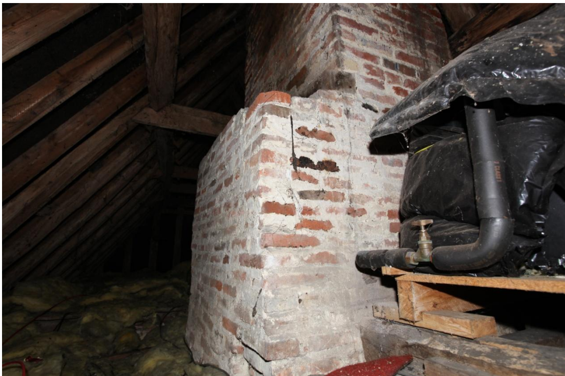
Illus. 22. The brickwork of the chimney exposed in the roof space showing its thick mortar and irregular bricks in the typical manner of the 17 th century. The upper courses and external stack were rebuilt in uniform soft reds with fine mortar joints in the 19 th century.
