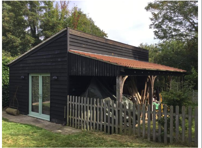
Photo 2 South-east elevation of Studio 1
