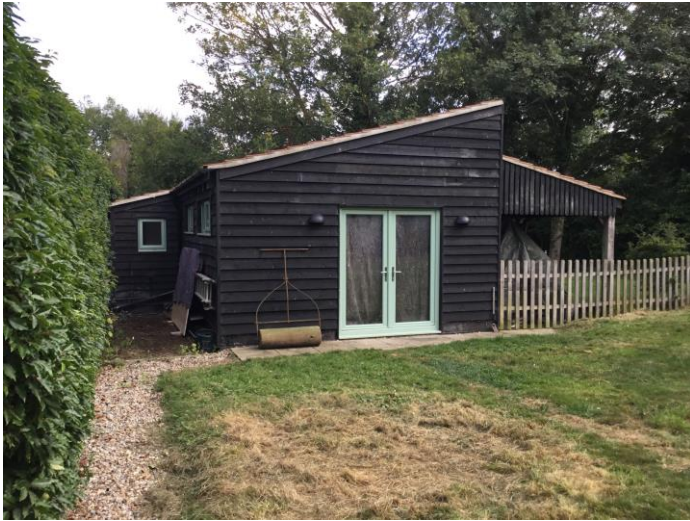
Photo 1 South-west elevation of Studio 1
