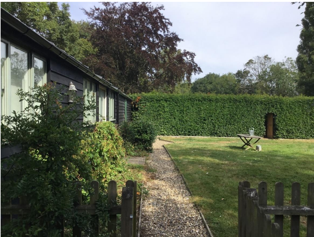
Building 1 – front elevation from left hand end
