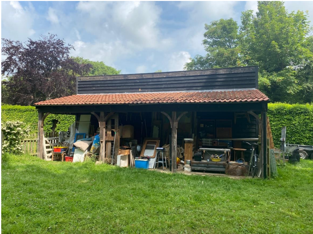
Building 2 – right side showing lean-to addition
