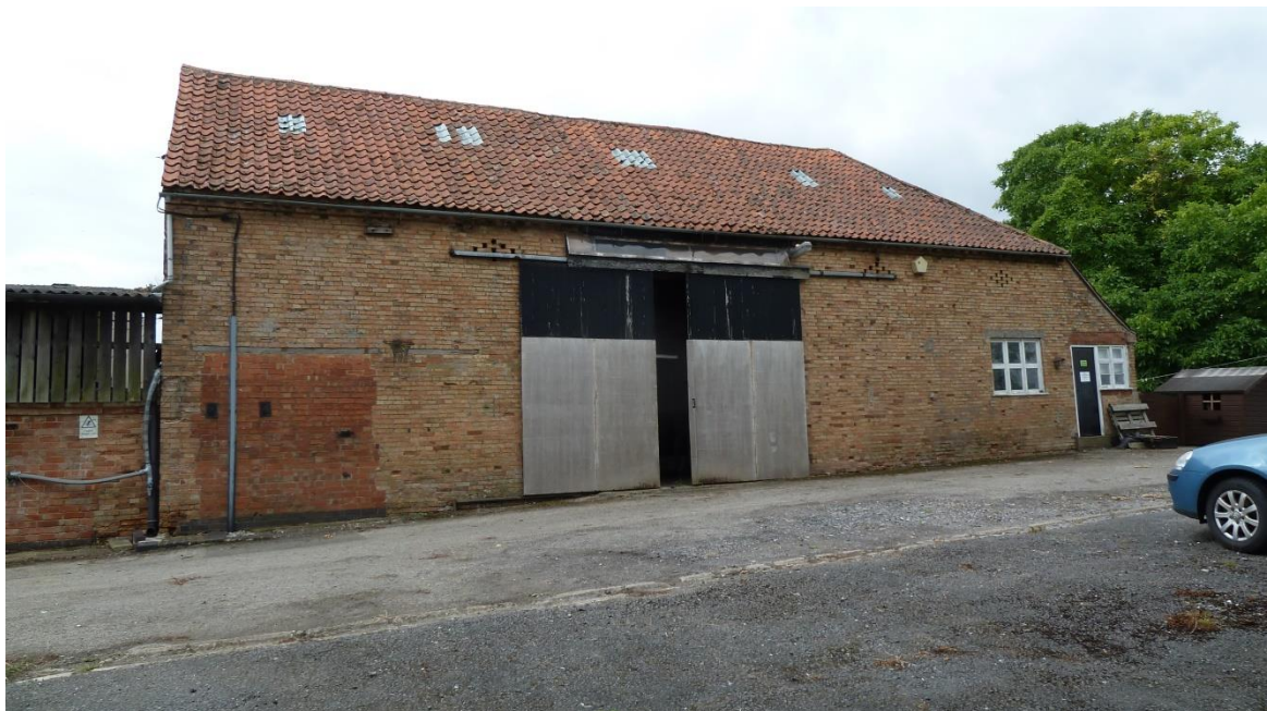
Photograph 1 – Building 3, two-storey solid brick barn.
