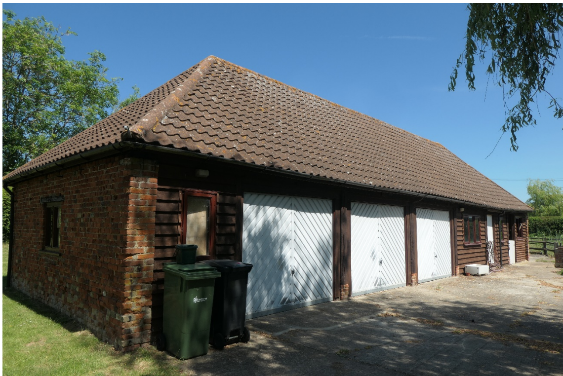
Photo 8 , south and west aspects of the garage on site.
