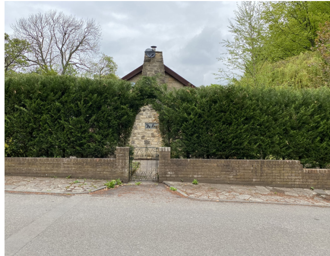
Fig 02 - View from North Lodge towards application property
