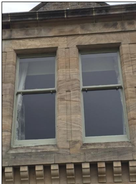
Photo 4. The old first floor sash windows
