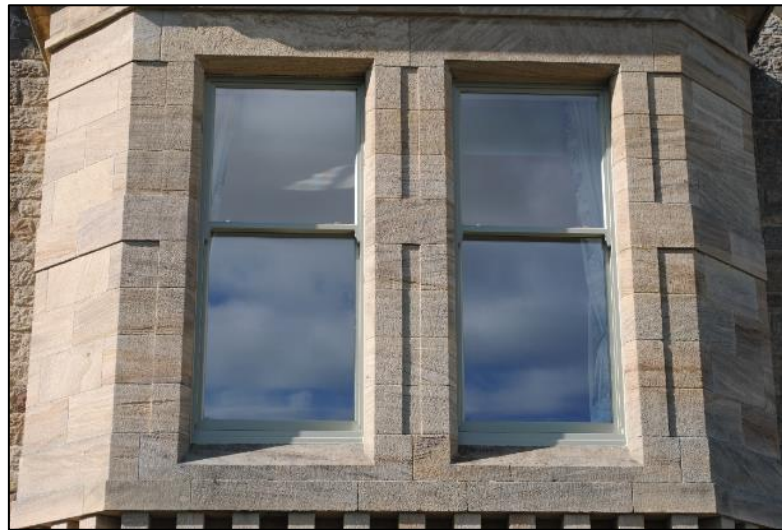
Photo 7. The replaced first floor sash windows
