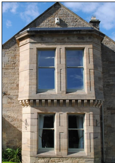
Photo 8. Traditional and replacement windows
