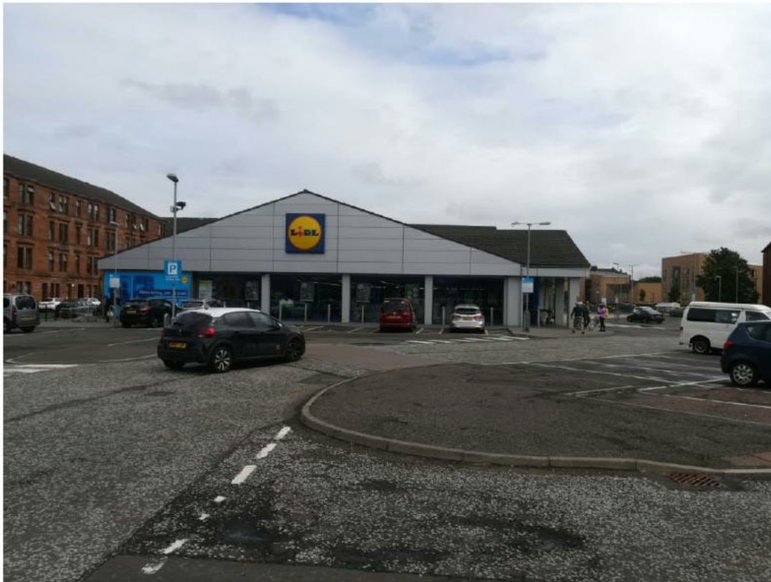
Photo 4: Front of Lidl building.
