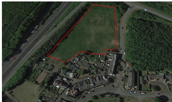
Figure 2: Google Earth Pro Image of Application Site and Surrounding Development
