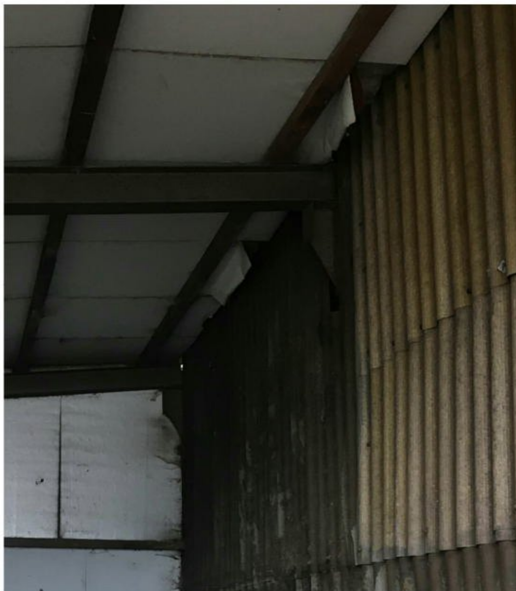
Figure 10: Lean-to support angle.
