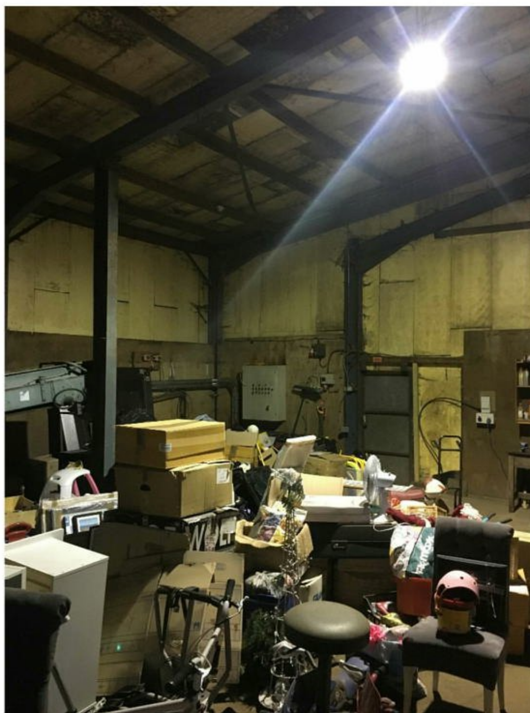
Figure 6: Incomplete roof bracing.
