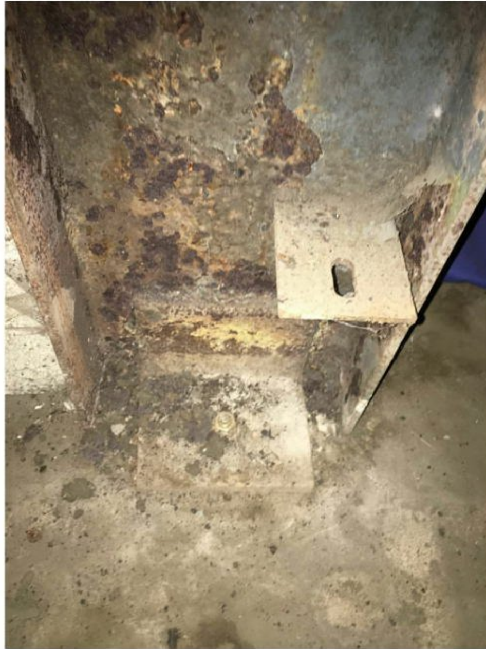
Figure 3: Internal column baseplate.
