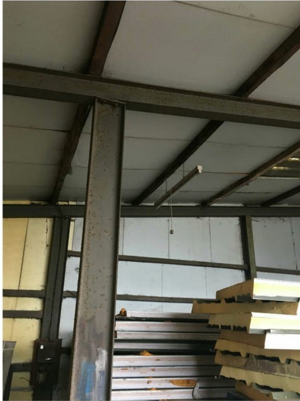
Figure 11: Column capping plate detail.
