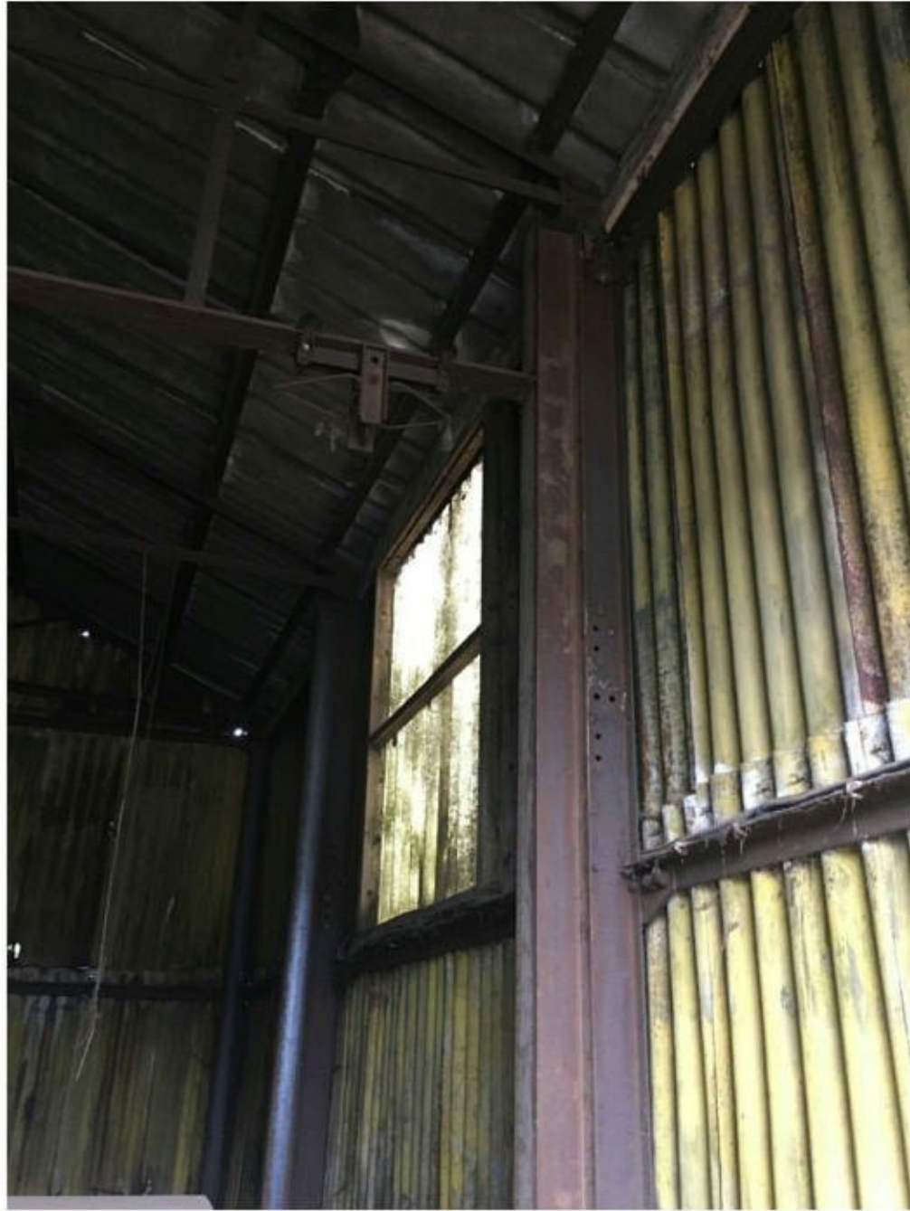
Figure 9: Rolled steel joist columns with retrofitted 152UBs.
