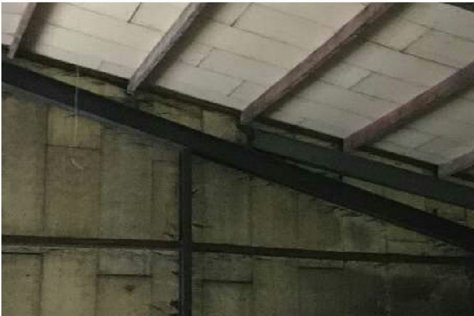
Figure 2: Steel connection to gable portal frame.
