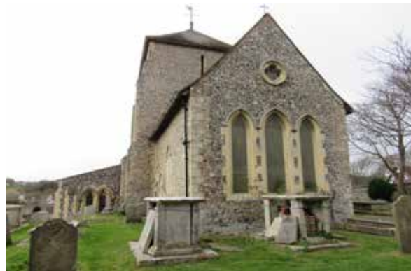
Figure 2.4 - The east elevation of St Margaret's Church.
