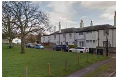
Figure 3.2 - Grade II Listed, 2 storey dwellings to the south of the site, looking south east
