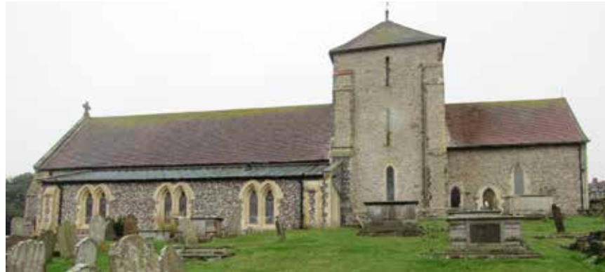
Figure 2.3 - The south elevation of St Margaret's Church.
