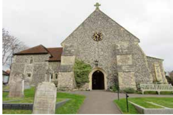
Figure 2.2 - The west elevation of St Margaret's Church.
