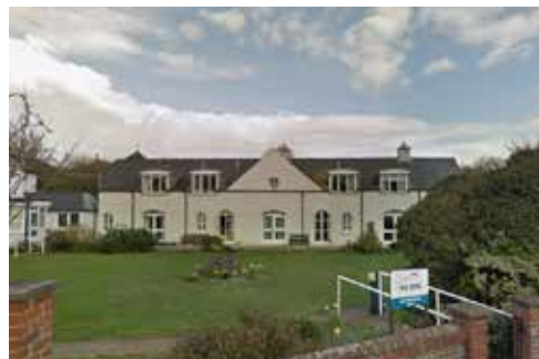
Figure 3.4 - Terraced properties at the Dene, a retirement village, looking east
