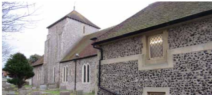
Figure 2.5 - The north elevation of St Margaret's Church.
