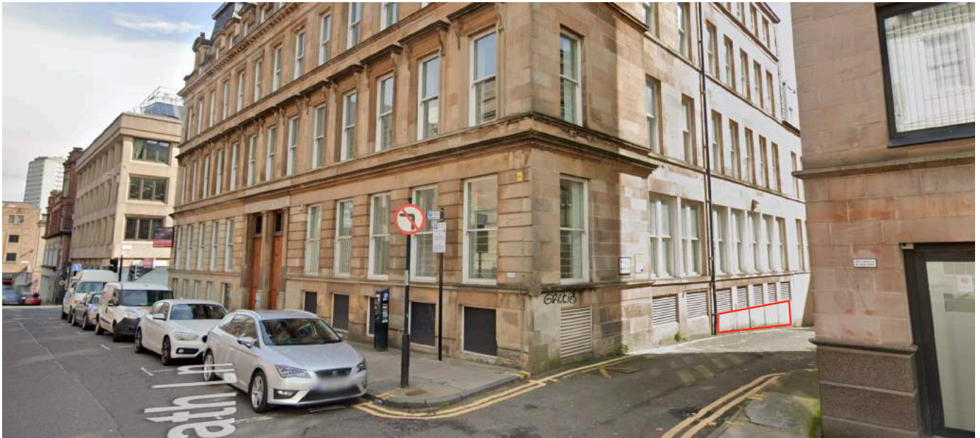
Figure 2 shows the location of this as viewed from Wellington Street. The additional louvres are designed to sit within the existing pilasters, with the existing openings cut down to provide the additional ventilation space required. The client is proposing to paint these louvres to match the colour of the surrounding stone, as has been done with those that are existing in order to reduce their visual impact.
