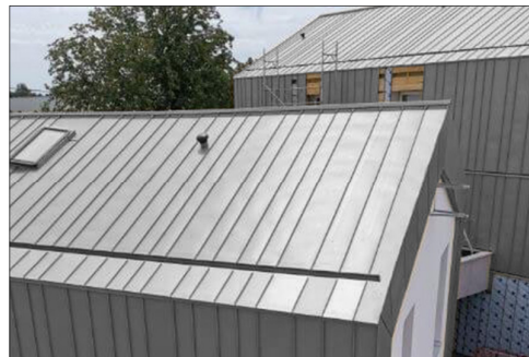
Zinc Roof Cladding
