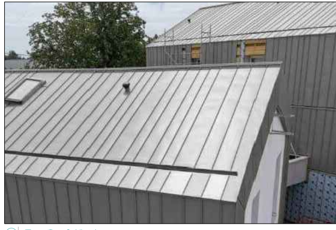
① Zinc Roof Finish Varied Width Cladding
