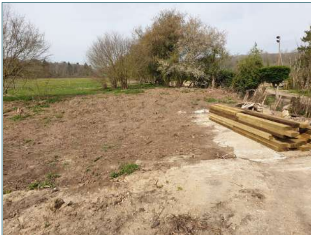
Photograph 3. Area within the Site for the proposed dwelling footprint.
