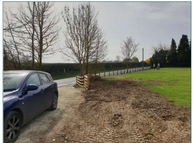
Photograph 4. Existing access from Maidstone Road, comprising crushed hardcore.
