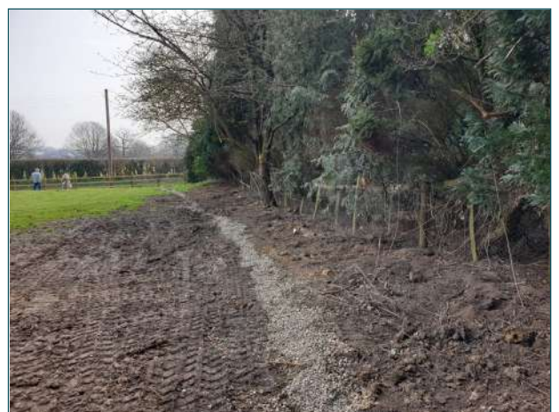
Photograph 6. French drain in southern portion of the Site.
