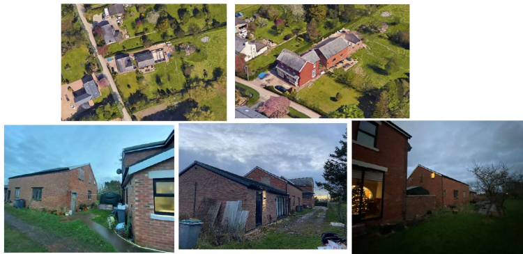
Site photos from visit carried out 15/12/2020 as part of previous application
