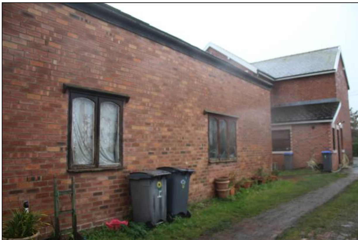
3. The outbuilding has rebuilt walling and modern windows
