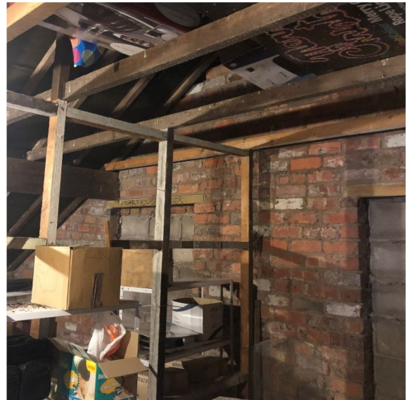
Photograph 5: Internal view of the eastern side of the barn.
