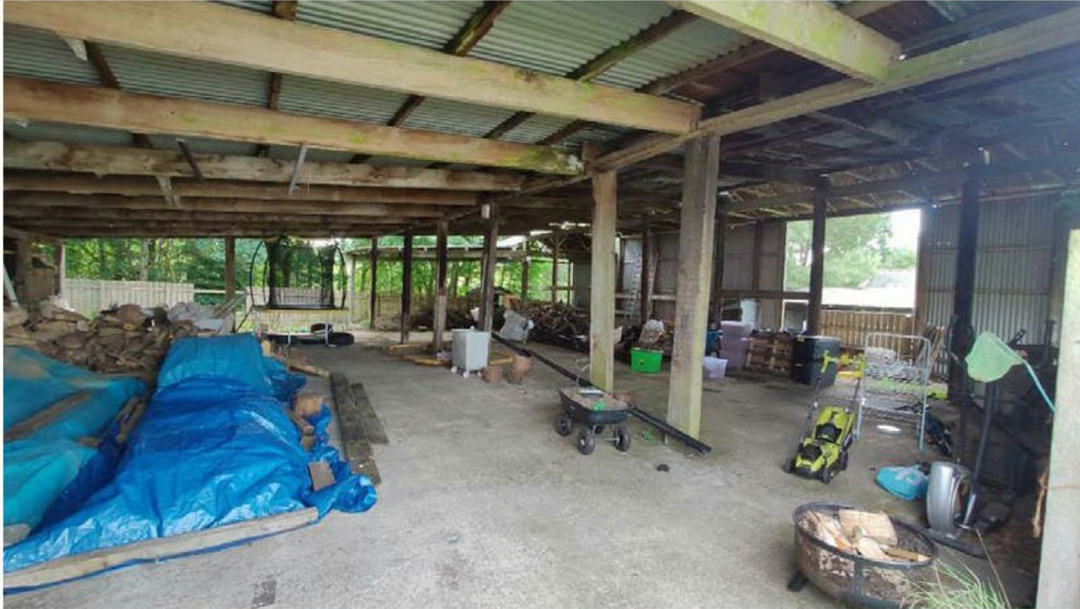
Photograph: 3 Showing example of usage within eastern former agricultural barn
