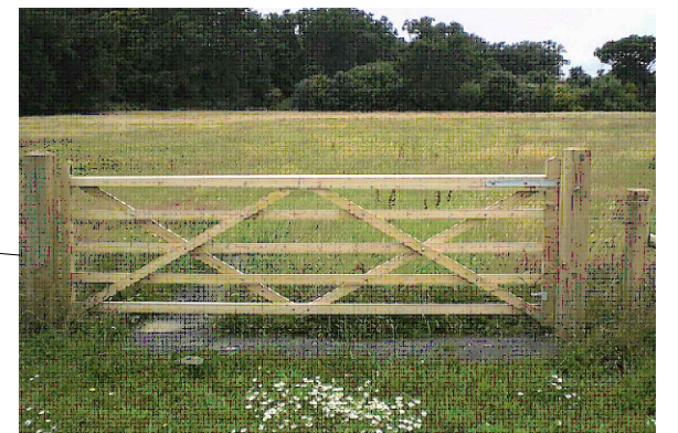
FIVE BAR WOODEN GATE AND POSTS TO ENTRANCE
