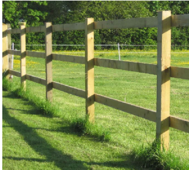
TREATED TIMBER POST AND RAIL FENCE
