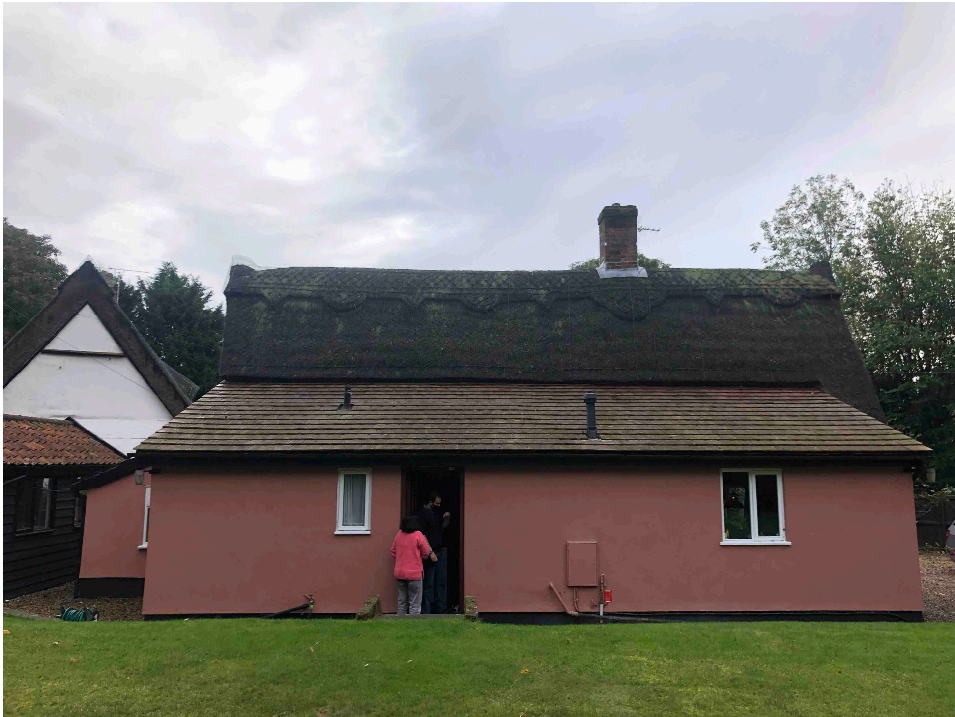
Rear view of modern lean to. Width of new extension to match but thatch restored as modern lean to roof removed. The restoration and reinstatement of the thatch is a significant enhancement
