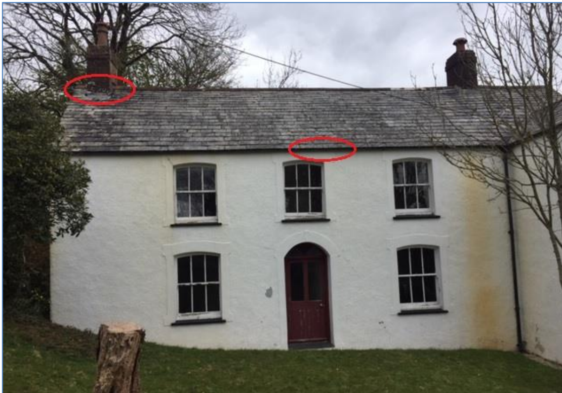
Fig 4 – Bat emergence points – south elevation.
