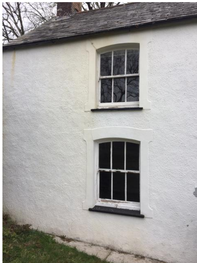
Fig. 10: Part South elevation, showing the extent of historic materials and methods of construction that are to be retained as part of the proposals. It is proposed that the timber sash windows are to be replaced; however, the profiles and materials are to be replicated to match existing.
