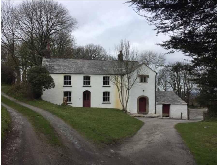
Fig. 5: View from South toward the South Elevation of the dwelling with the unmade driveway leading down to the primary entrance of the dwelling. Single Storey coal shed to the right of the image attached to the East elevation of the dwelling.
