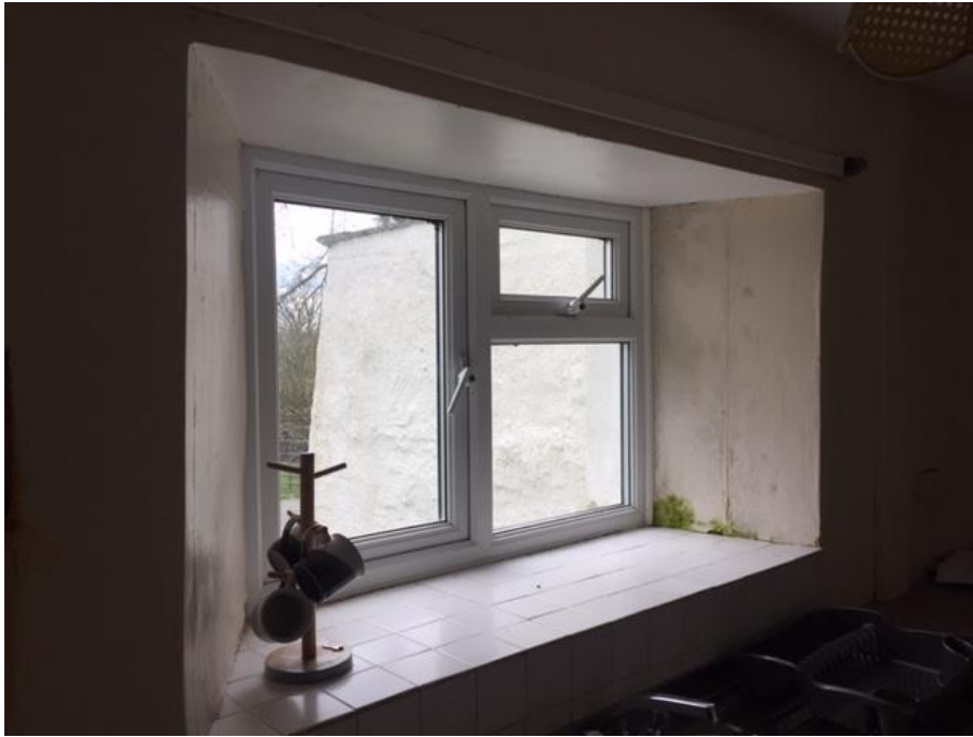
Fig. 9: The existing Kitchen window that shall become an extended to floor level to form a new doorway that will be the new entrance into the utility and downstairs shower room. Note modern UPVC window to be removed.
