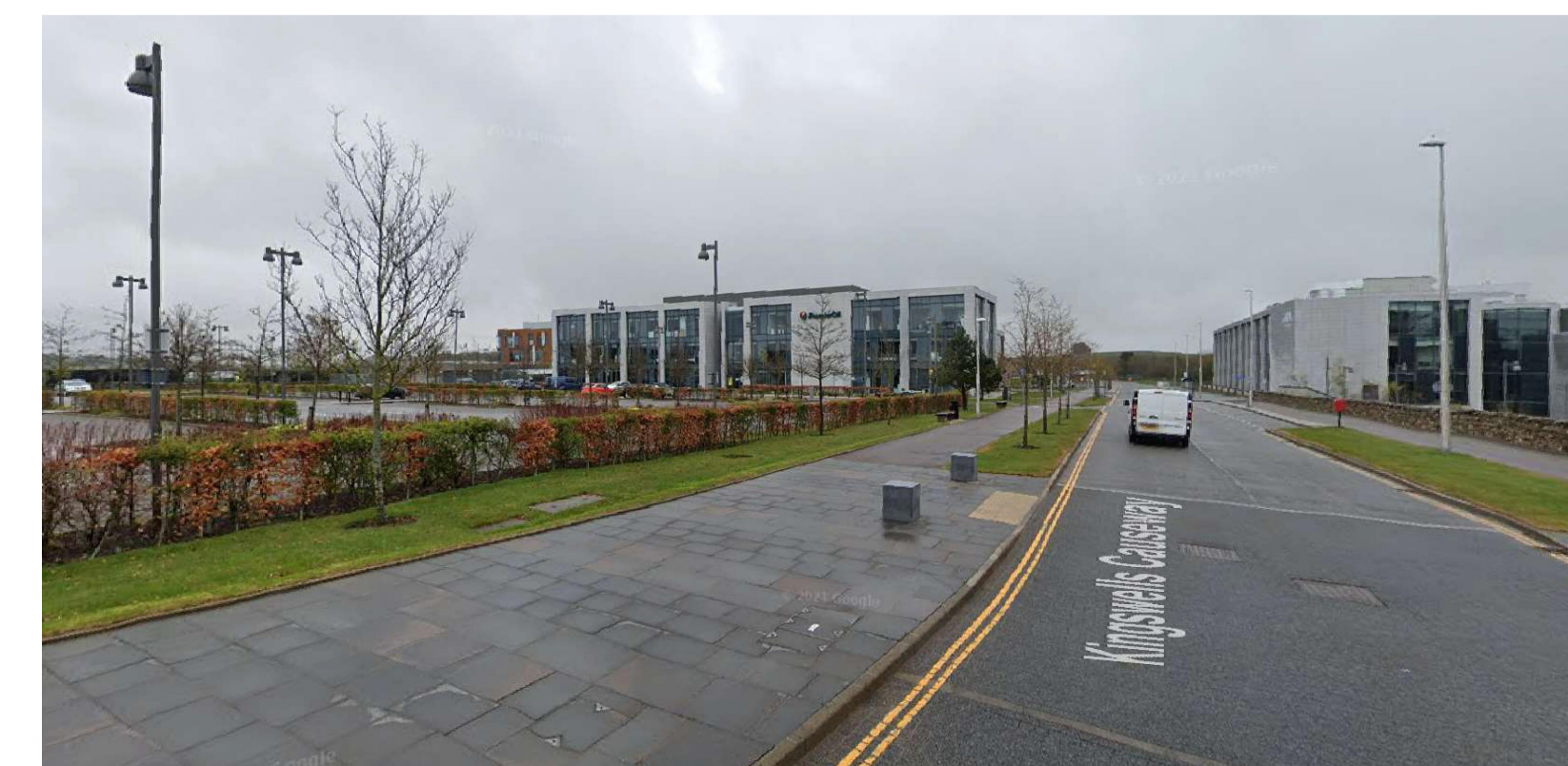
EXISTING VIEW LOOKING EAST
