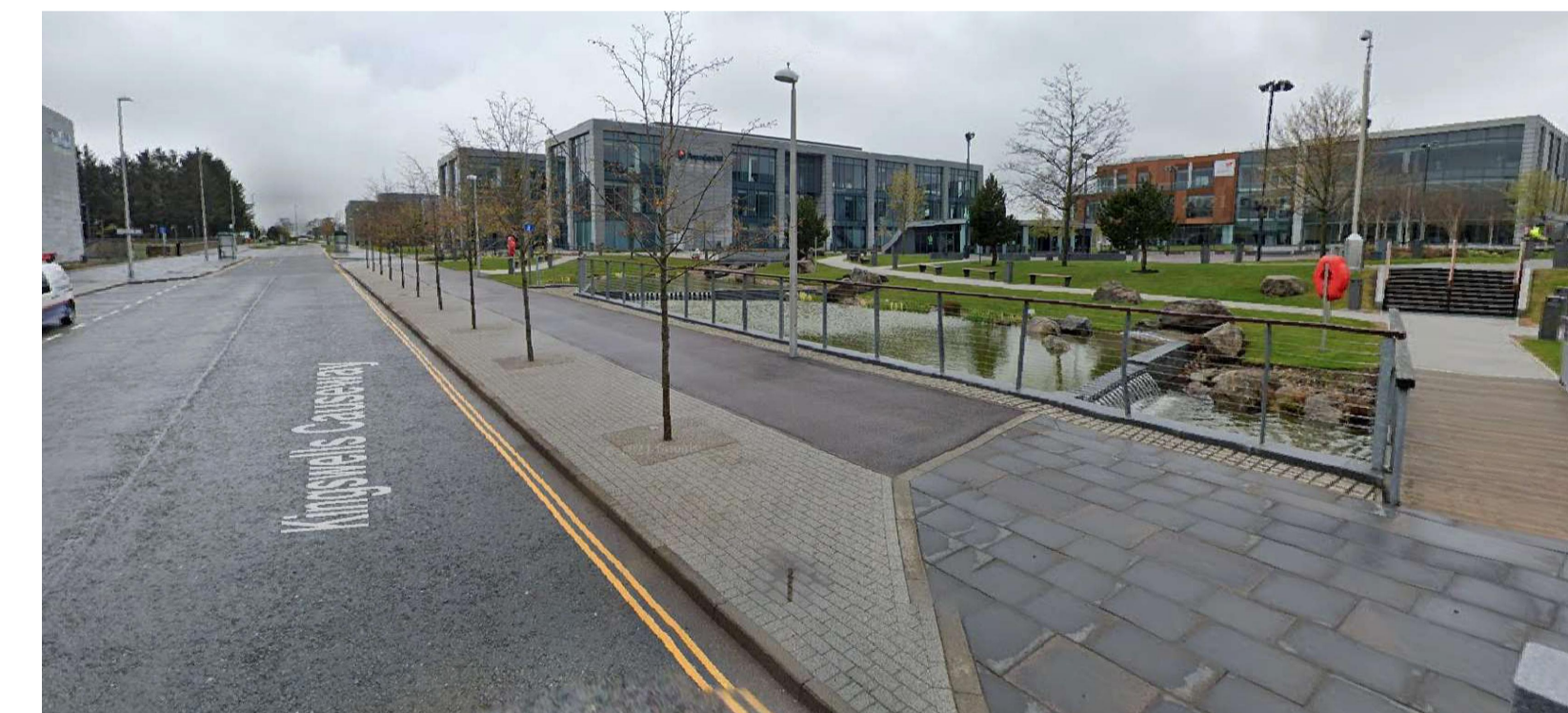
EXISTING VIEW LOOKING WEST
