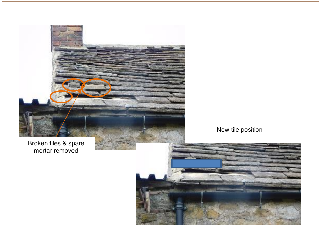
Figure 16 – New tile position
