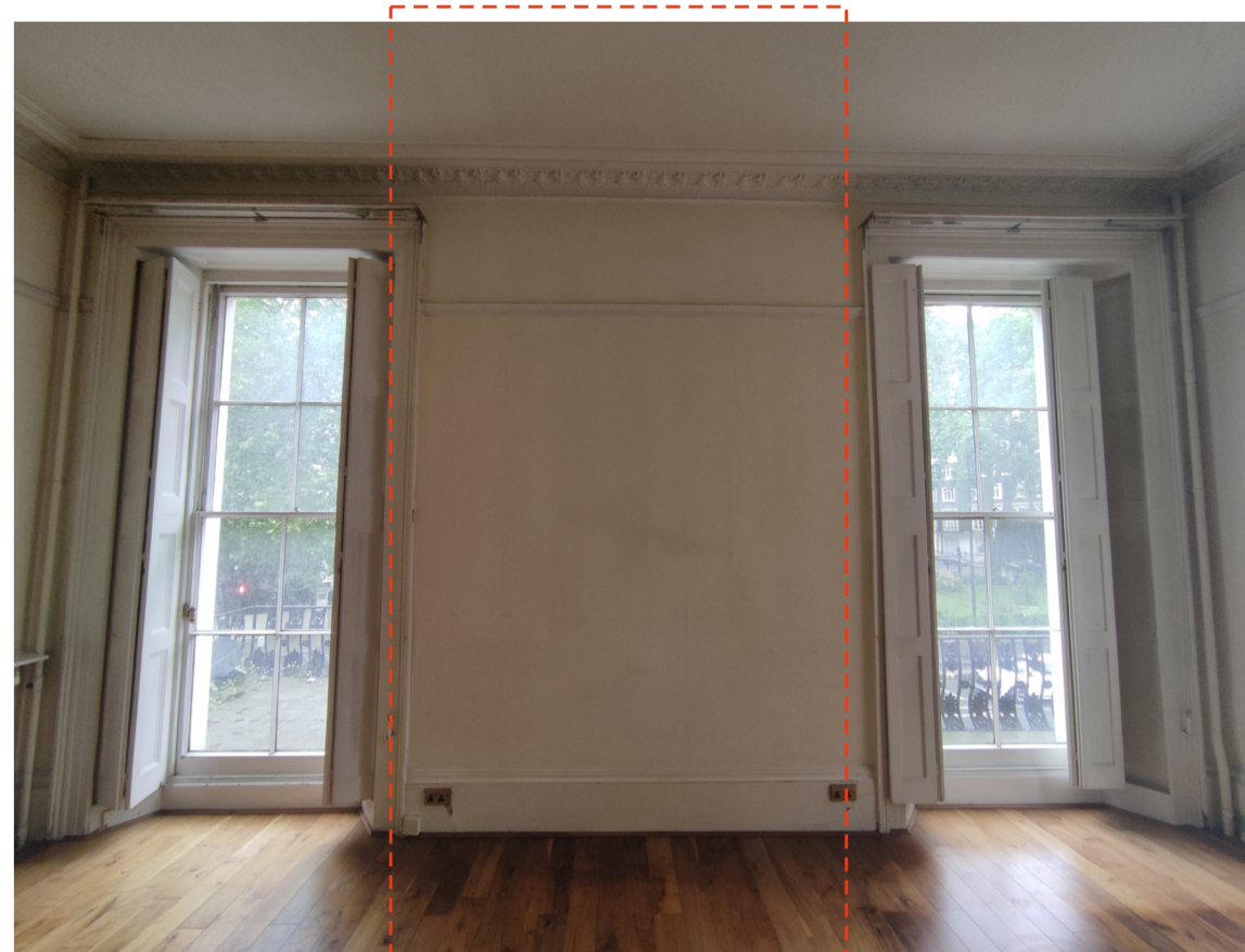
Photograph of Existing Internal Elevation. Red block denotes location of new window.
