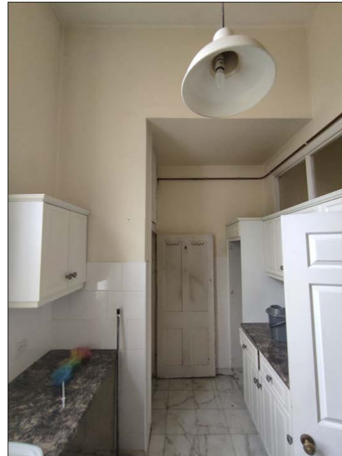
View B - Existing kitchen area. New dropped ceiling to rear of kitchen to be removed and original height to be reinstated. Kitchen ceiling is at original ceiling height.
