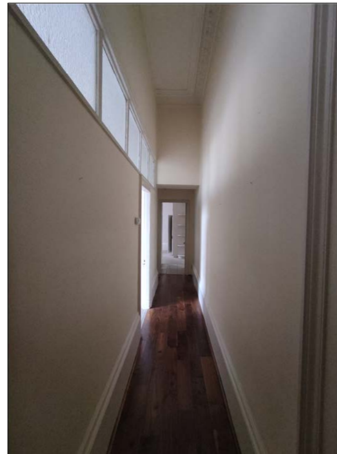
View D - View down entrance corridor New dropped ceiling beyond to be removed & ceiling level to be taken back to original and original room depth to be re-instated. Existing non loadbearing wall with clerestorey to be replaced with new. New glass clerestorey to run from top of new door opening to underside of ceiling allowing original volume and corning to be revealed
