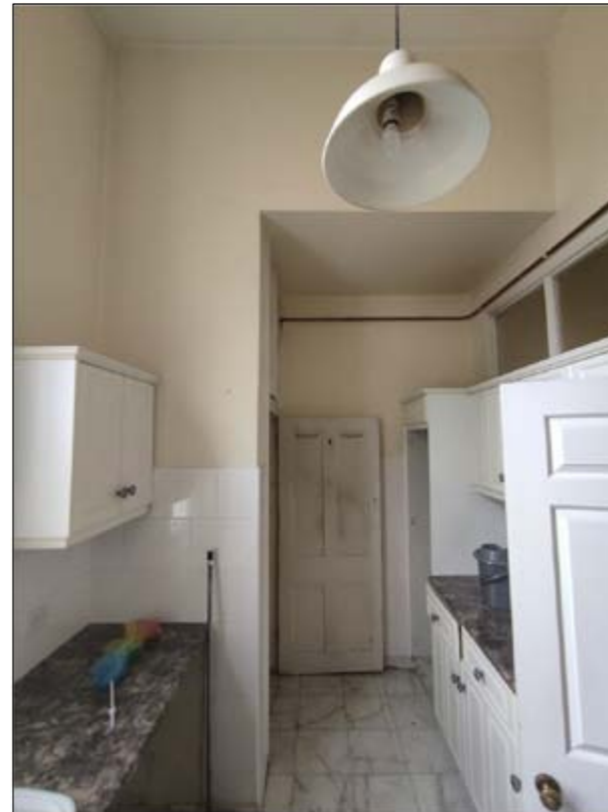
View B - Existing kitchen area. New dropped ceiling to rear of kitchen to be removed and original height to be reinstated. Kitchen ceiling is at original ceiling height.
