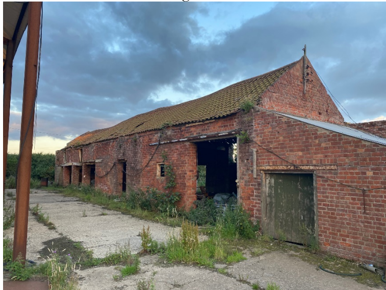
Plate 5 – barn 3 west gable and north elevation.
