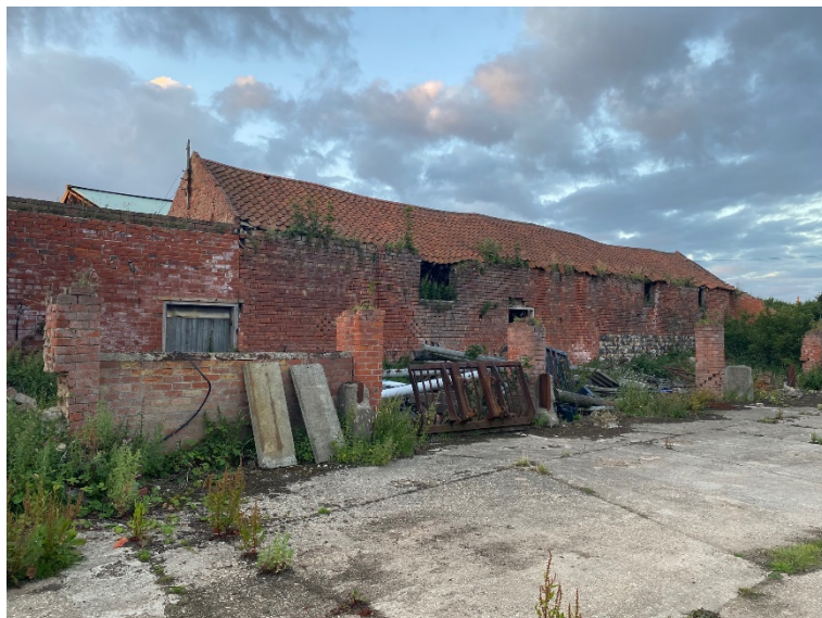
Plate 6 – barn 3 south elevation.
