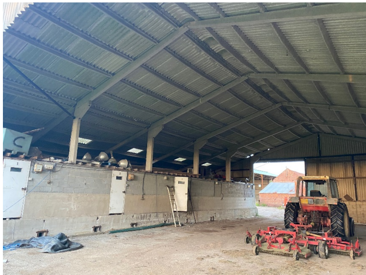
Plate 3 – barn 1 internal roof void.
