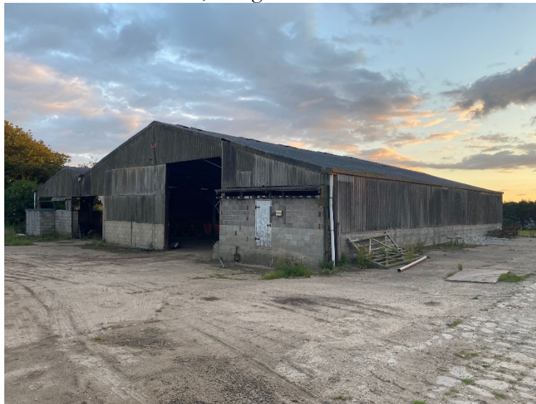
Plate 2 – barn 1, east gables and north elevation
