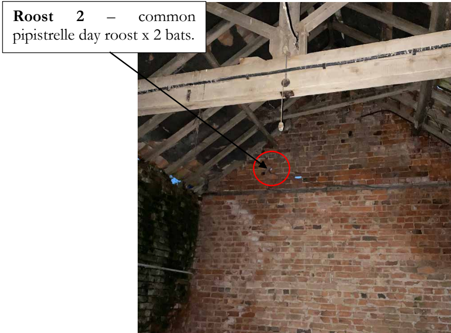
Plate 8 – barn 3 internal roof void.
