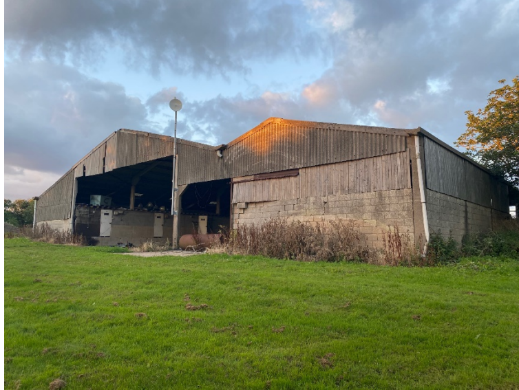
Plate 1 – barn 1, west gables and south elevation
