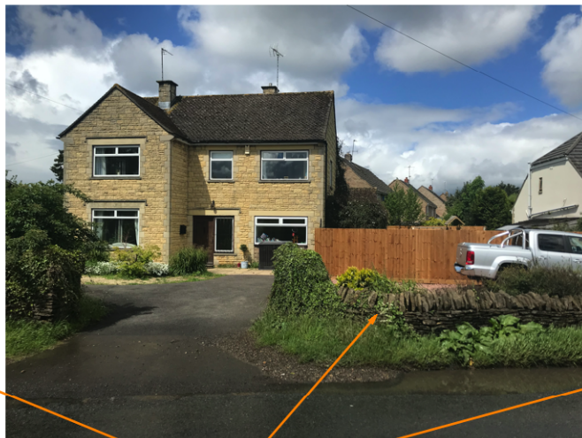
EXISTING 800-900MM DRYSTONE WALL WITH COCK & HEN COPING
