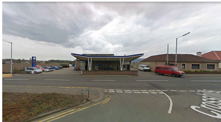
VIEW FROM NORTH
