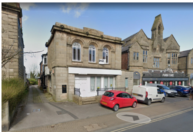
View looking east along Derby Street.
