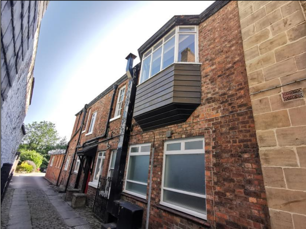
Plate 4 – Side with access road, west facing elevation
