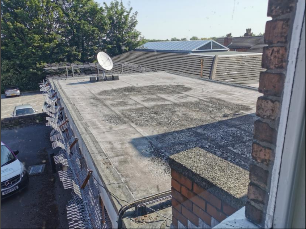
Plate 7 – View of the flat roofs proposed for removal
