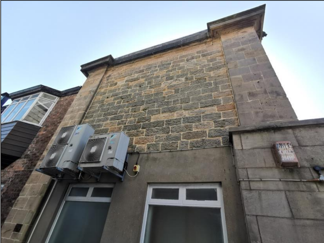
Plate 6 – Side with access road, west facing elevation stone segment
