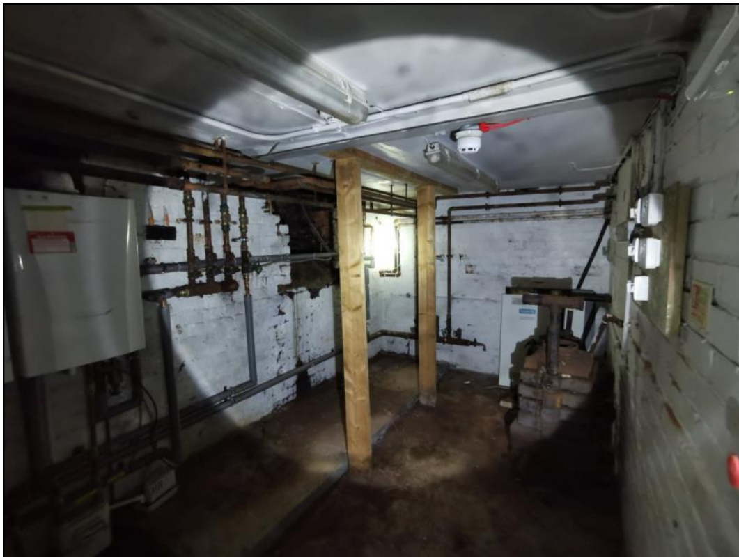
Plate 15 – Cellar of the former bank section
