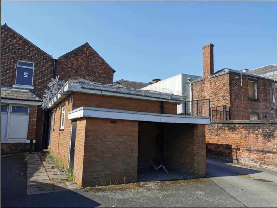
Plate 3 – Rear with car park, north facing elevation, alternative
