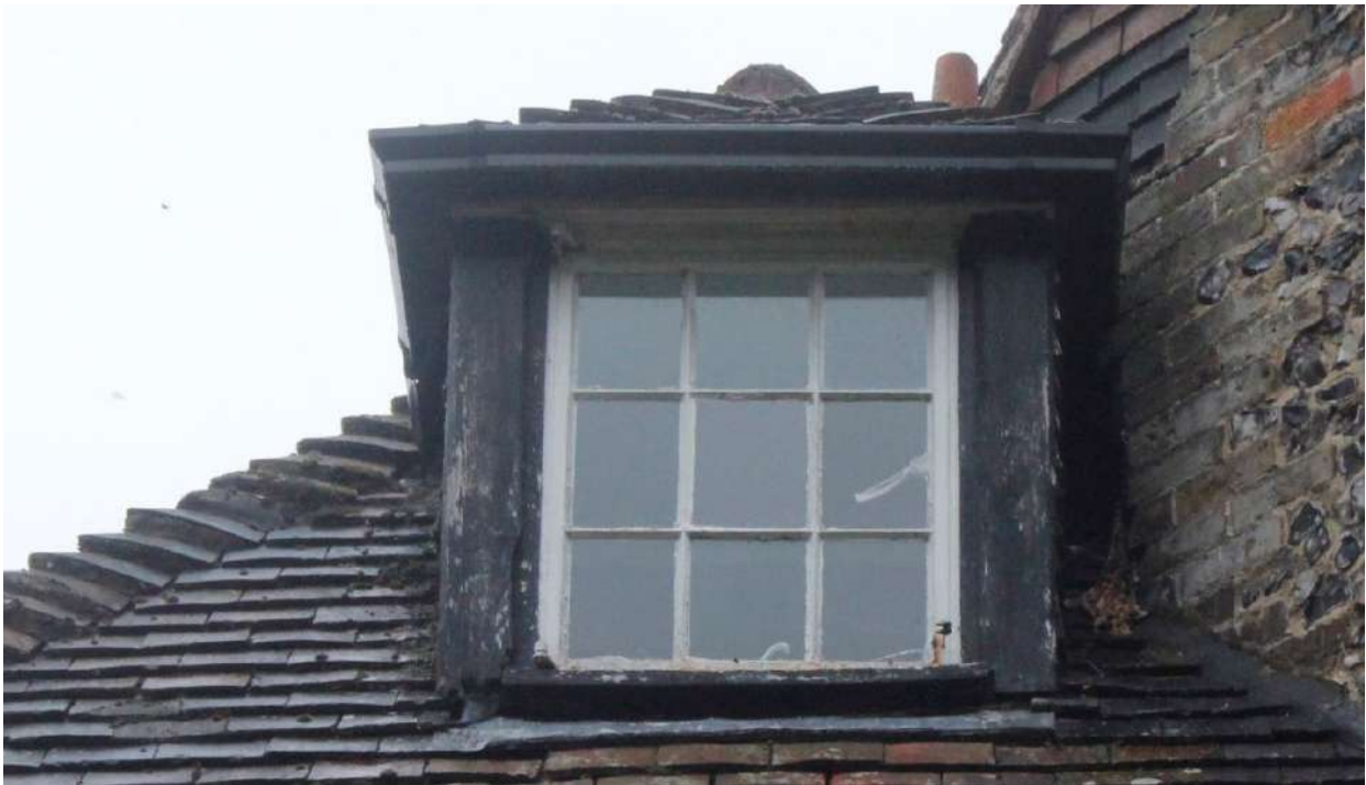
Window 95 – hidden behind tree – Crittall
