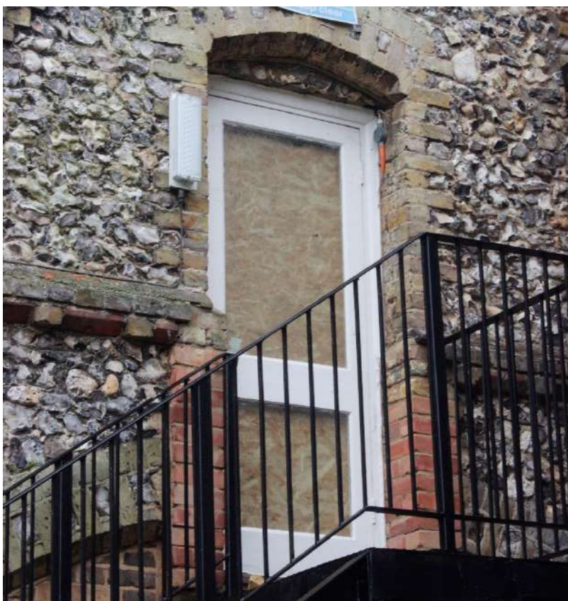
Window 62 – First floor wooden door to be replaced with a Crittall window
