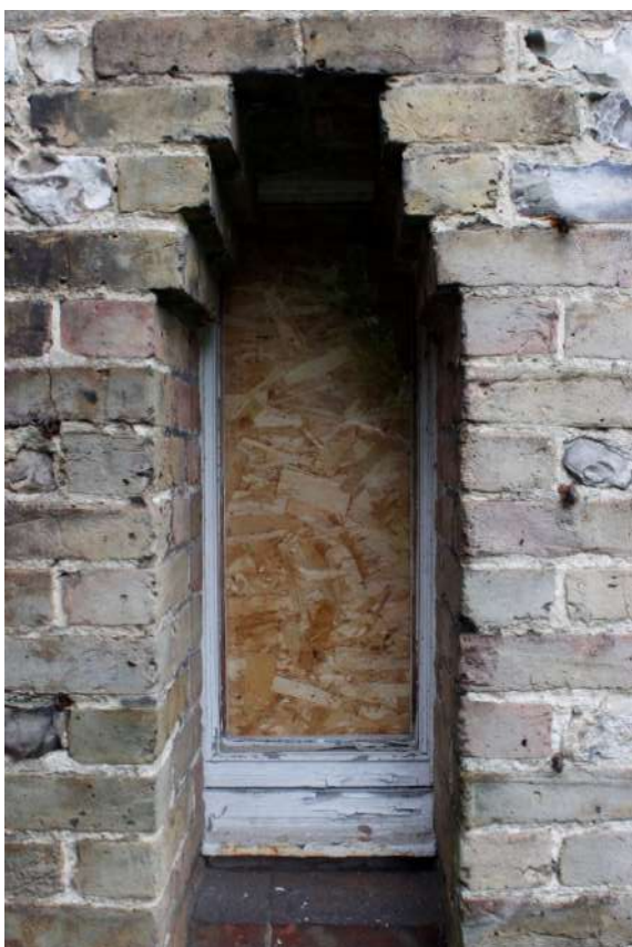
Window 62 – First floor wooden door to be replaced with a Crittall window
