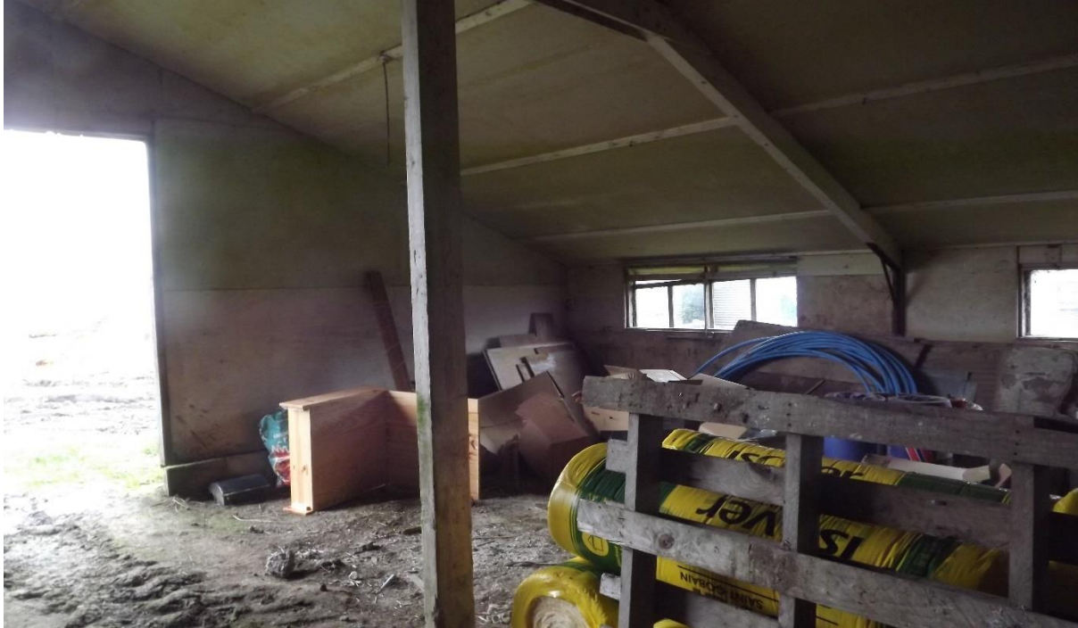
Photo 2. Asbestos corrugated roof
