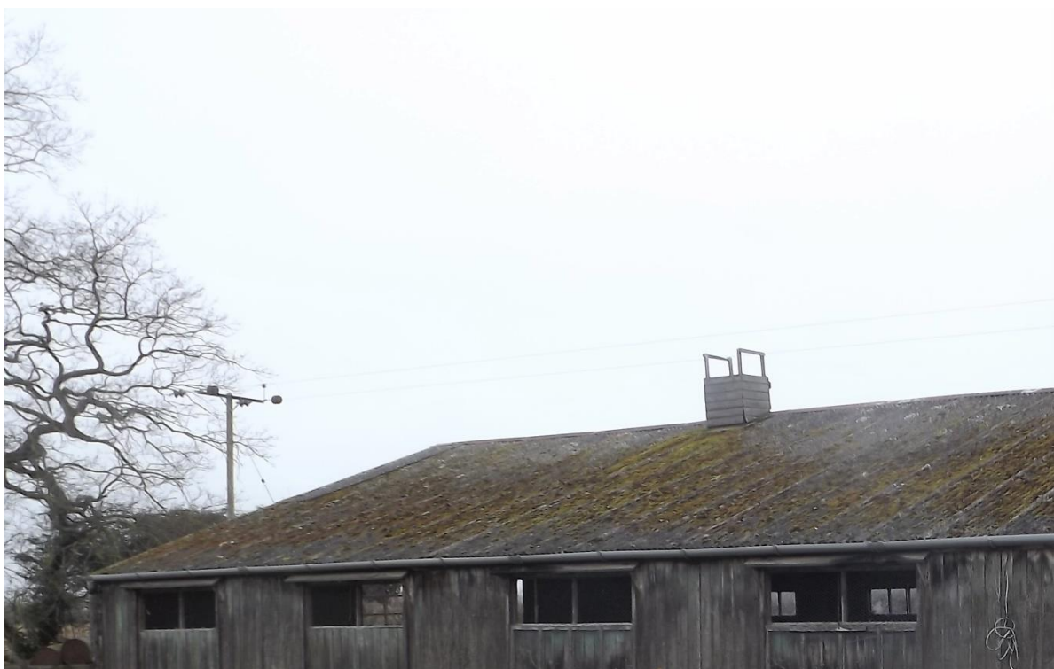
Photo 2. Asbestos corrugated roof
