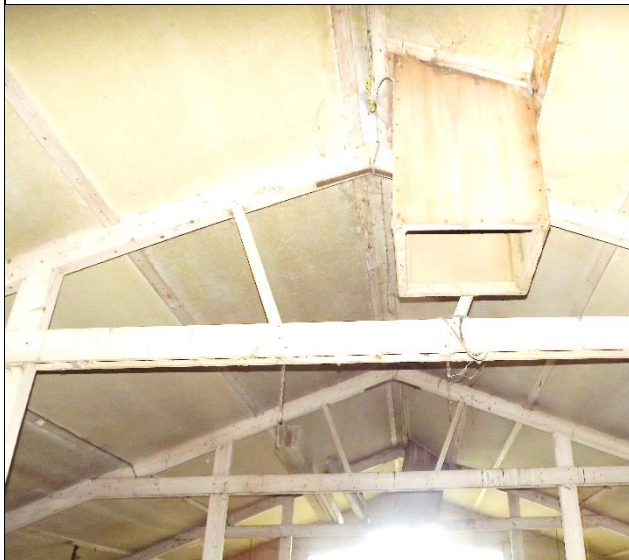
Bottom left: Timber rafters with fire boards.
