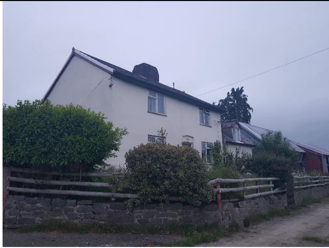
South west facing gable end.
