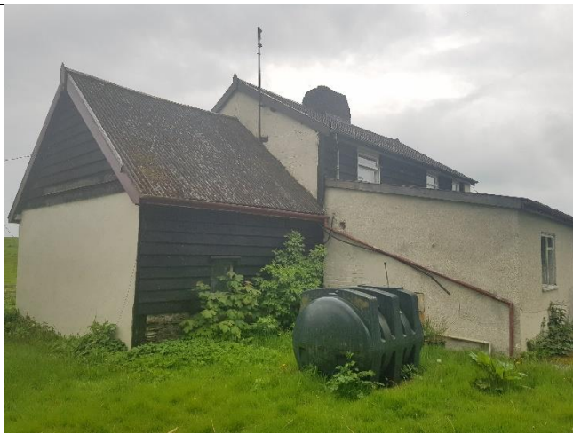
North east facing gable end.
