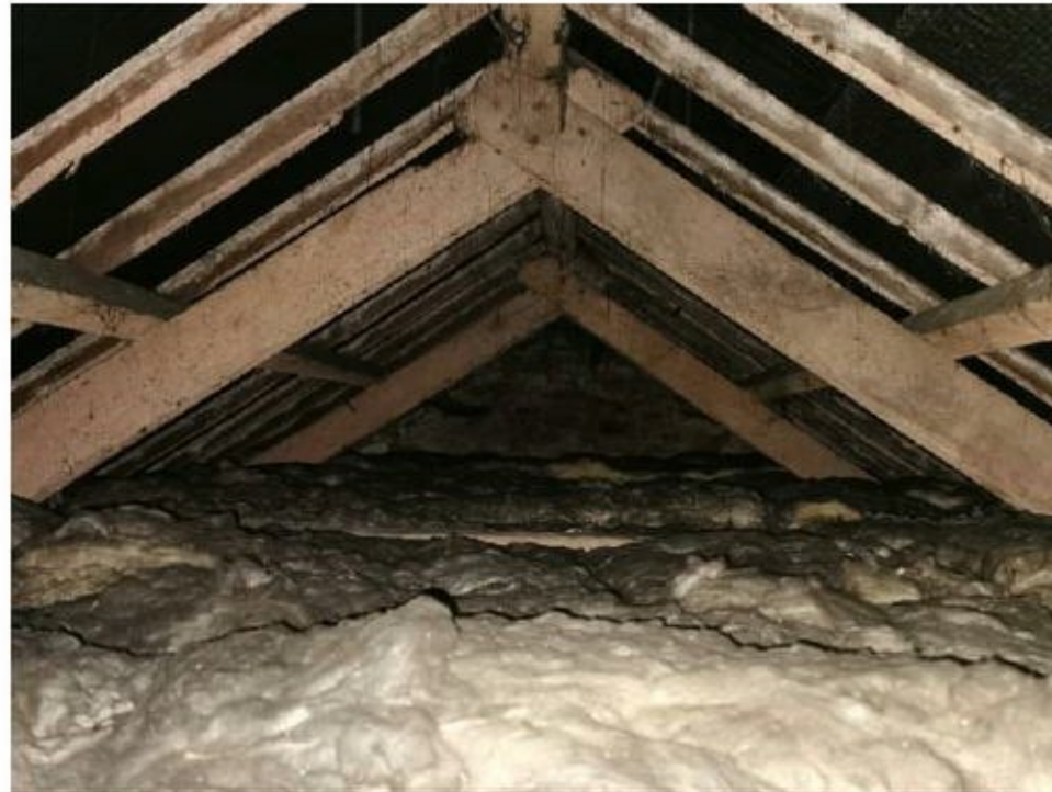
Photos 4. Showing the roof void over the house
