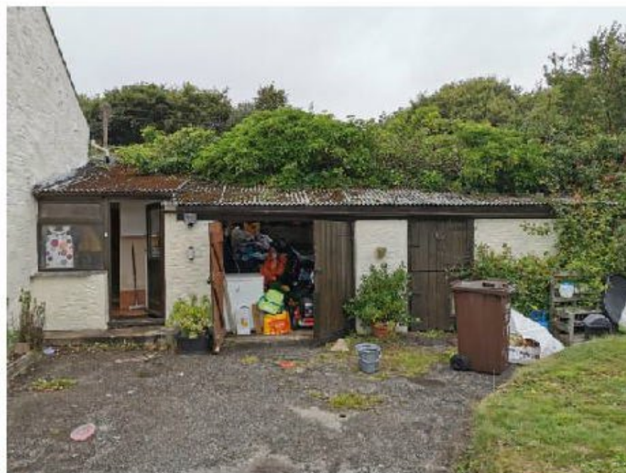
Photo 3. Showing the attached stable block
