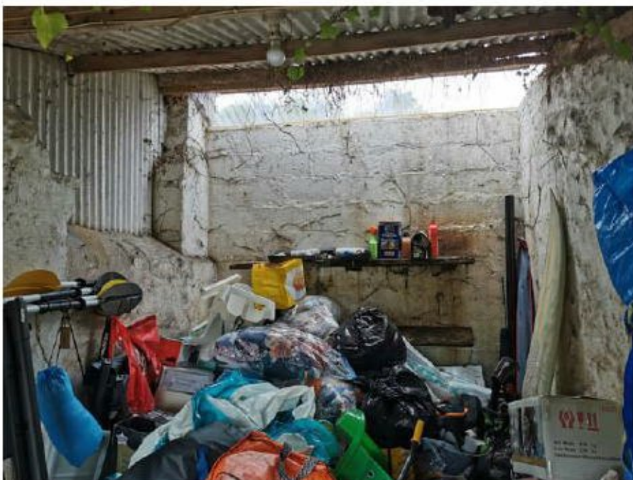
Photo 5. Showing the central room in the stables
