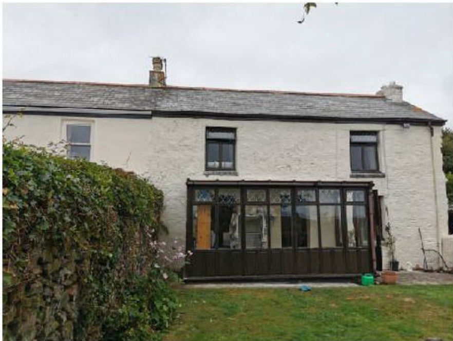
Photo 1. Showing the house from the south
