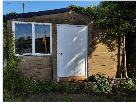
Image 4. Prefabricated concrete shed
