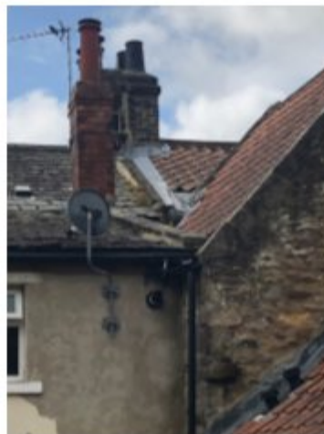
Brick chimney stack to be removed with valley gutter
